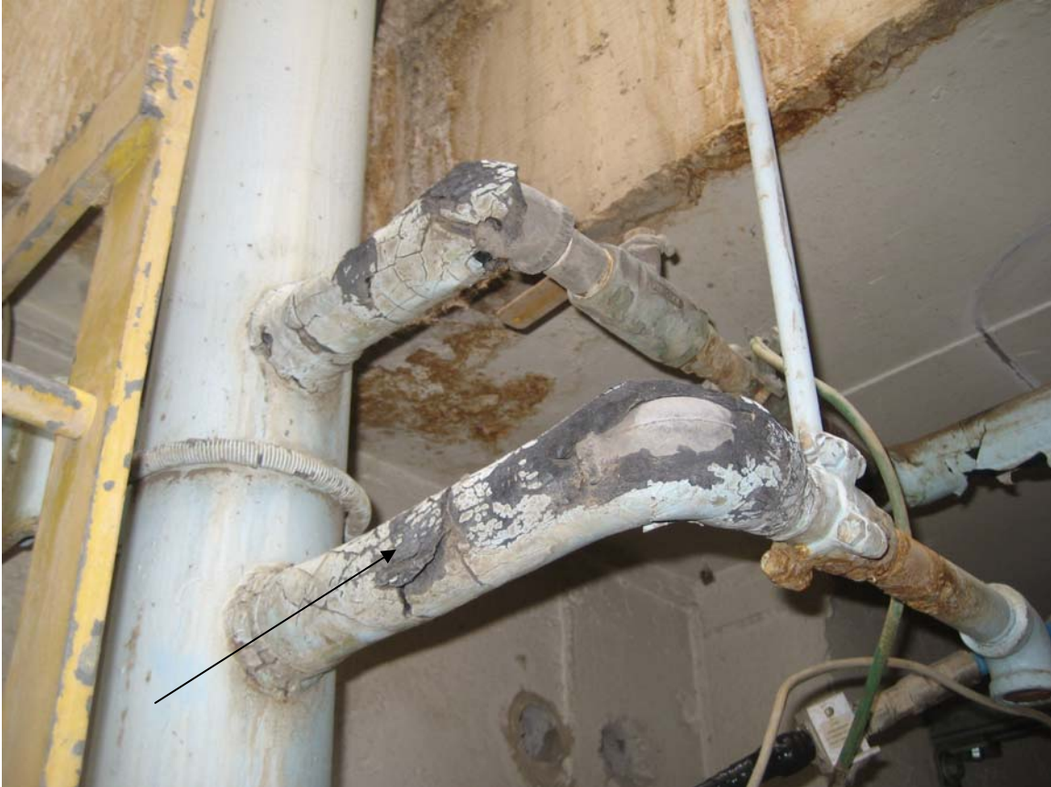
HA #11 – Non asbestos containing black pipe covering
