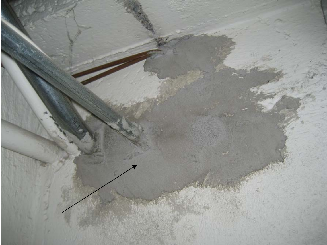
HA #9 – Non-asbestos containing wall penetration fireproofing
