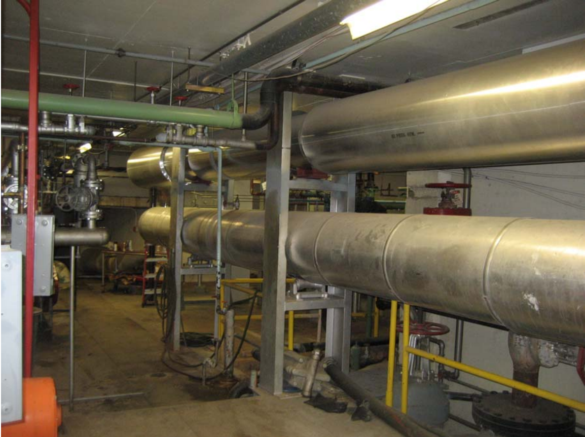
HA #6 – Assumed asbestos containing 12”-36” metal jacketed steam line insulation
