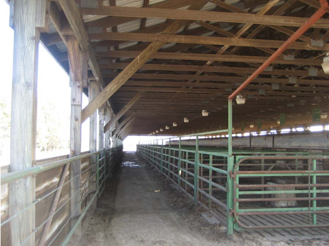
Interior View of Animal Shelter, Looking West
