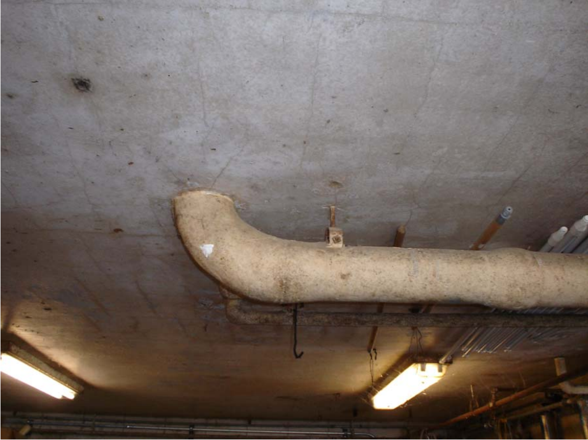
HA #7 – Non asbestos containing canvas wrap on fiberglass pipe straight insulation
