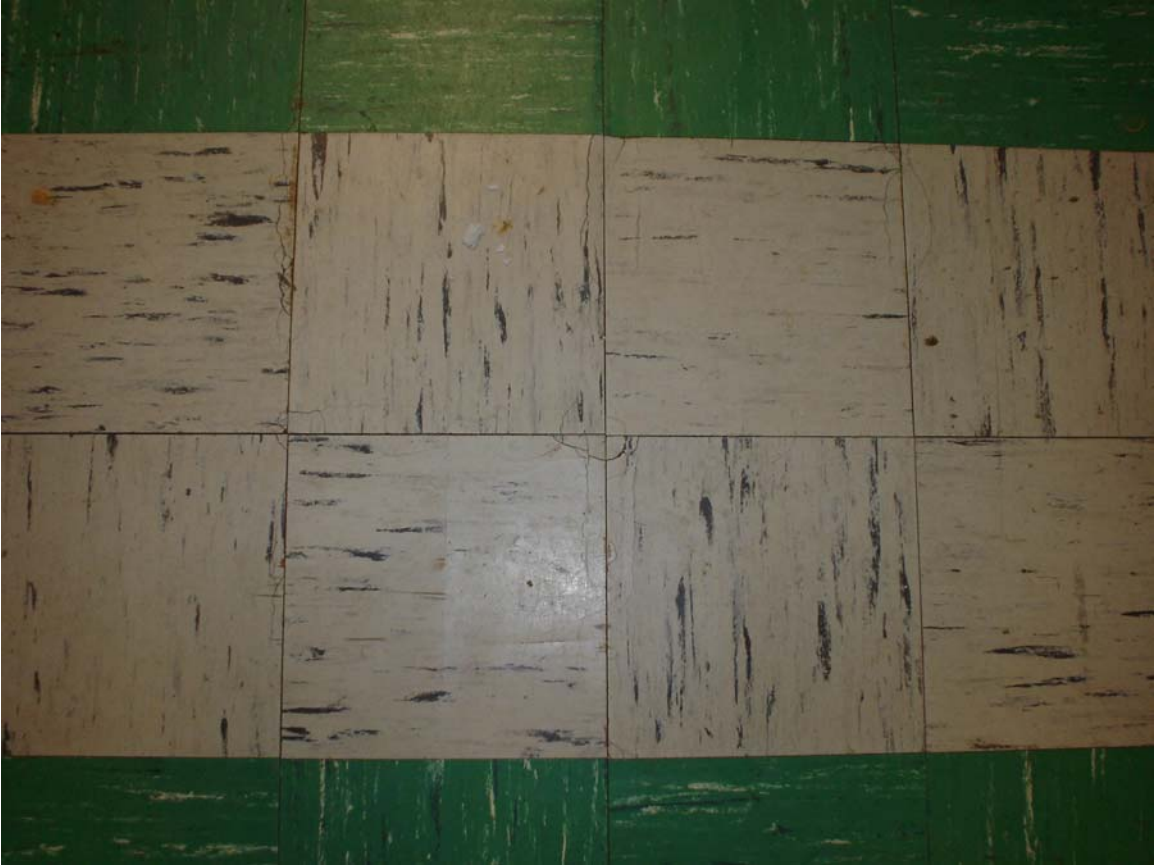
HA #2 – Non asbestos containing 9” x 9” white floor tile with black streaks and associated mastic
