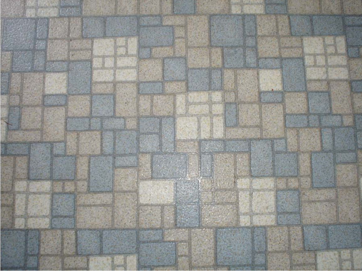
HA # 15 – Non asbestos containing multi-colored square pattern linoleum and associated mastic
