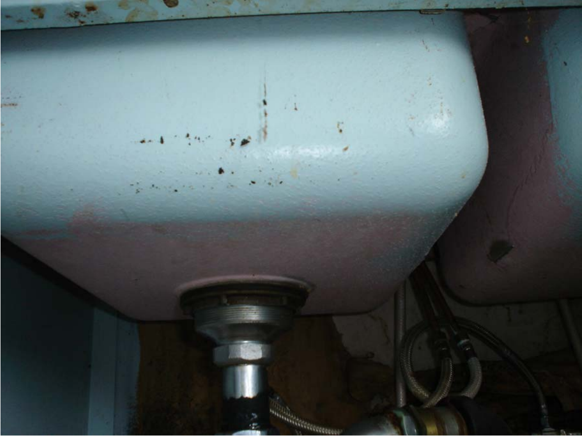
HA #14 – Non asbestos containing pink sink undercoating insulation
