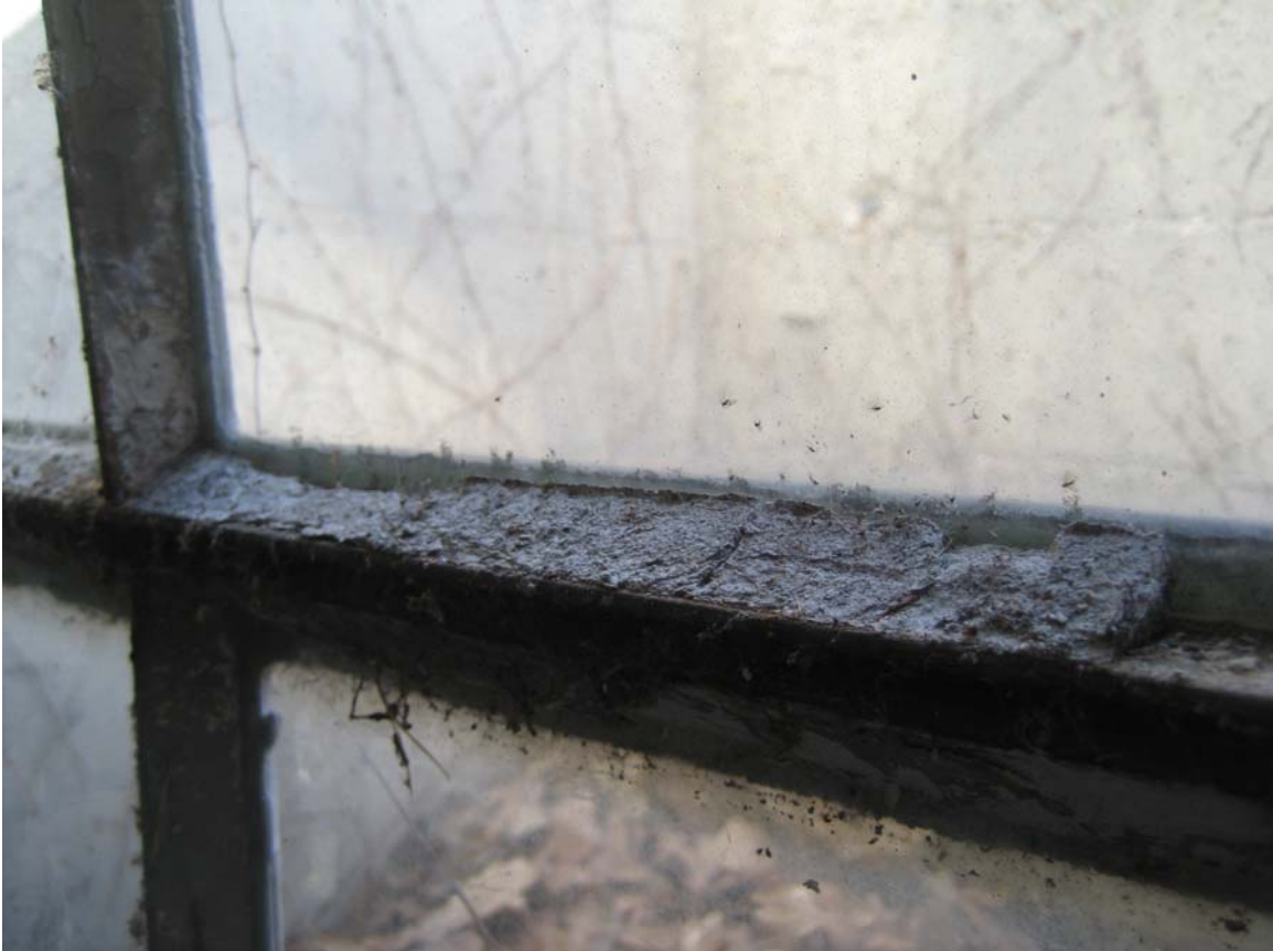
HA #2 – Asbestos containing white glazing compound
