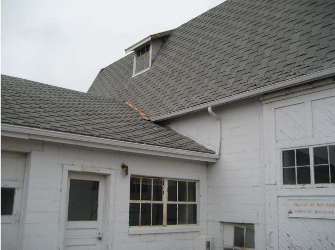
HA #12 – Non asbestos containing roofing materials (shingles)
