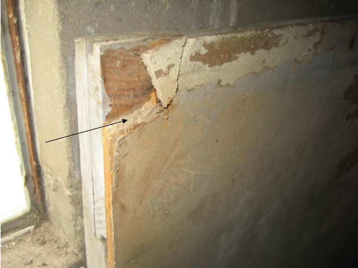
HA #6 – Non-asbestos containing drywall on wood, unfinished
