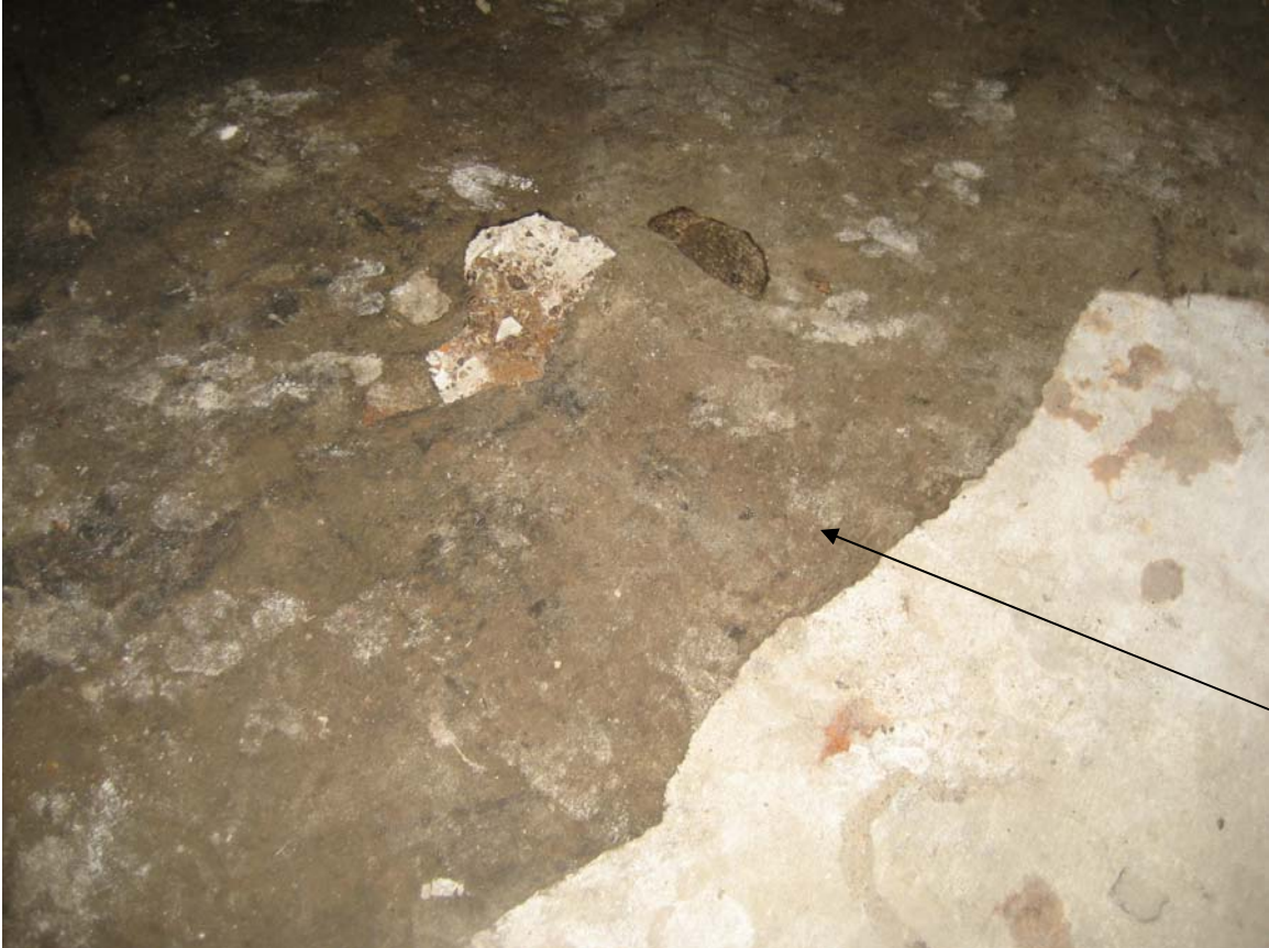
HA #7 – Non asbestos containing seamless floor covering (canvas)
