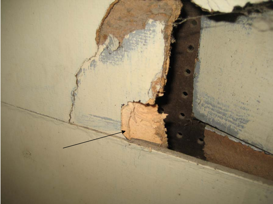
HA #1 – Non asbestos containing light brown wallboard and paper layer
