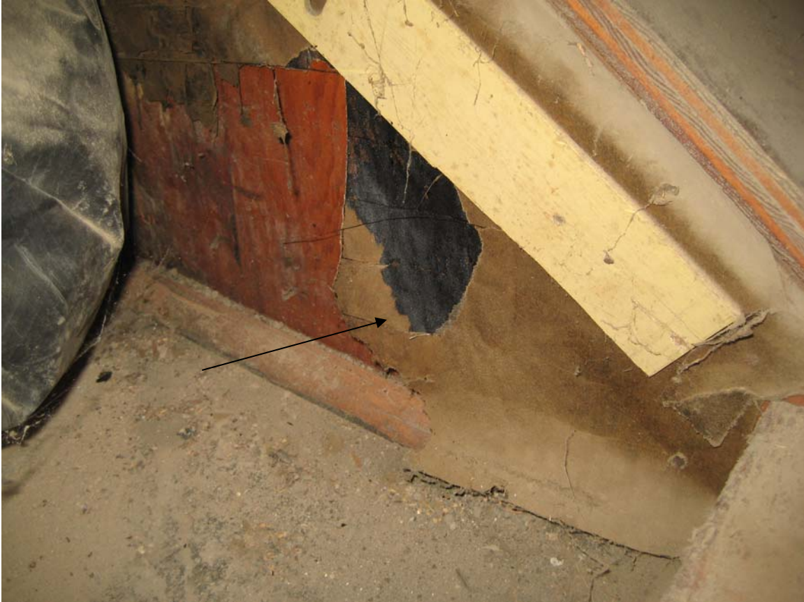
HA #10 – Non-asbestos containing brown paper with tar layer
