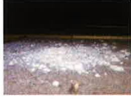
Picture #7--West Wing Room G-29 Basement
