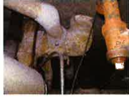
Picture #12--East Wing Room G-39 Basement
