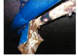
Picture #5--West Wing Crawl Space in G-25A Basement
