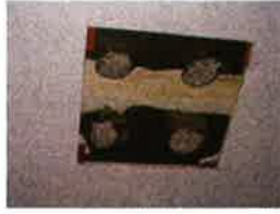
Picture #3--Central Section Center Hallway First Floor
