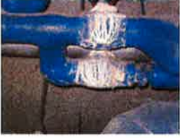
Picture #11--East Wing Mechanical Room G Base...
