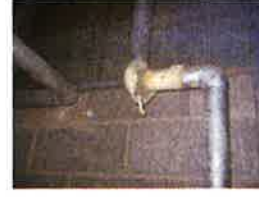
Picture #9--East Wing Room G-41 Basement
