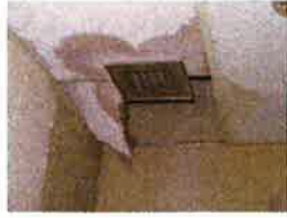
Picture #2--Center Janitor's Closet First Floor
