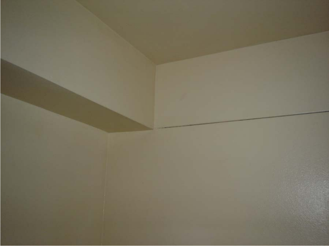
Asbestos-containing plaster
