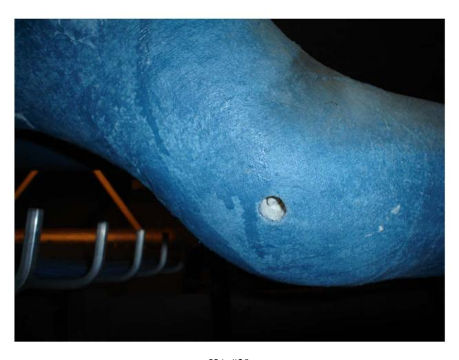
HA #30 Asbestos-containing domestic water supply and return pipe joint and hanger insulation
