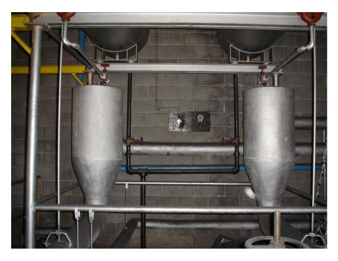
HA #48 Asbestos-containing silver expansion tanks
