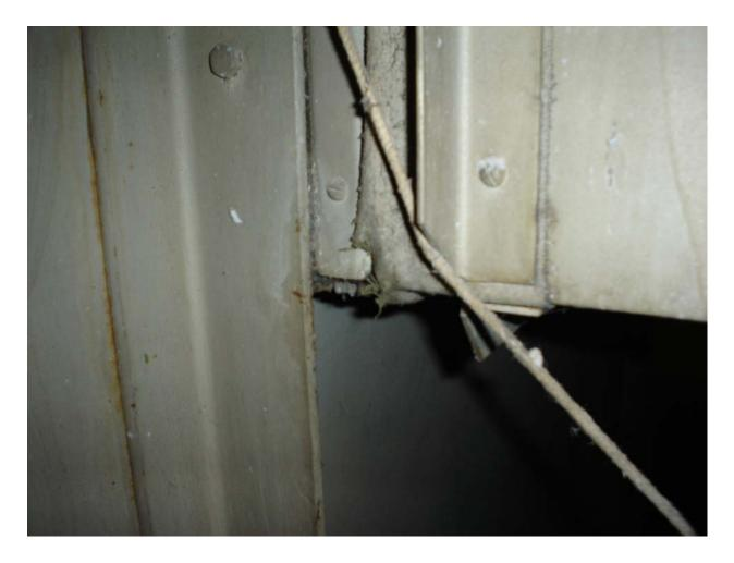
HA #34 Asbestos-containing white ventilation duct expansion cloth
