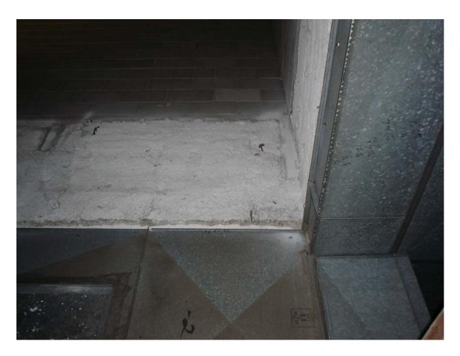
HA #40 Asbestos-containing spray-on fireproofing
