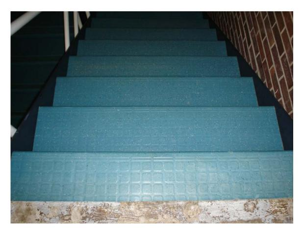
HA #13 – Non asbestos-containing green stair tread with cream and black specks and associated mastic
