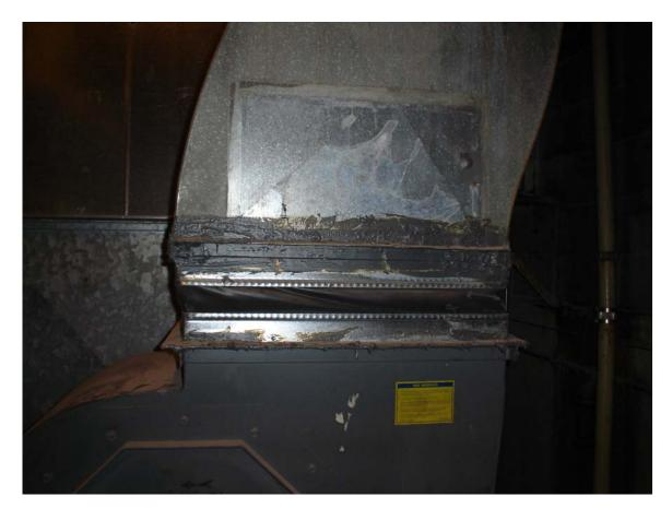
HA #6 - Non asbestos-containing gray HVAC duct caulk compound
