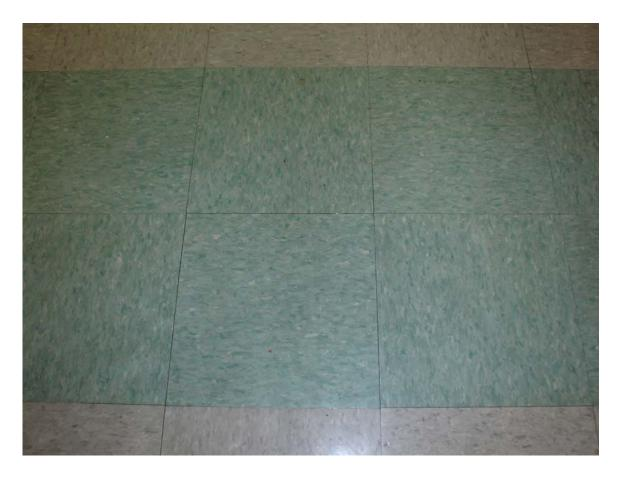
HA #22 – Non asbestos-containing 12" x 12" green floor tile with marble pattern and associated mastic
