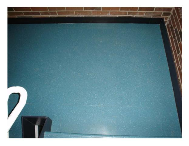
HA #12 – Non asbestos-containing 18" x 18" green vinyl flooring with cream and black specks and associated mastic
