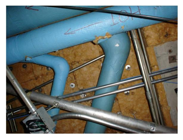
HA #4 – Asbestos-containing domestic water supply and return pipe joint and hanger insulation
