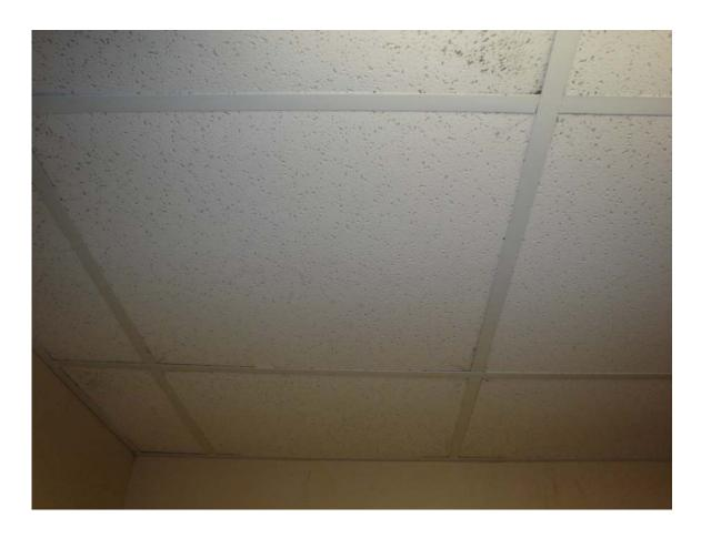
HA #37 – Non asbestos-containing 2' x 2' white lay-in ceiling tile with pin holes and fissures
