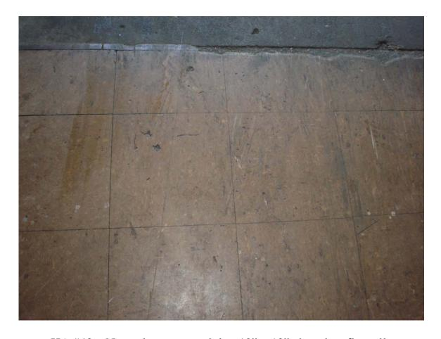
HA #40 – Non asbestos-containing 12" x 12" chocolate floor tile with yellow and rust streaks and associated mastic
