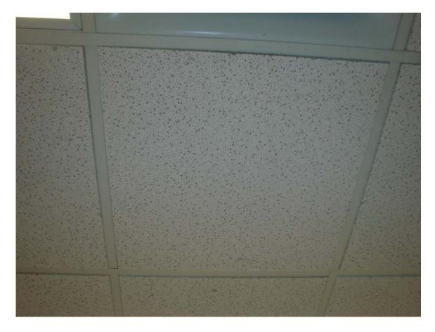
HA #38 – Non asbestos-containing 2' x 2' white lay-in smooth gypsum board ceiling tile
