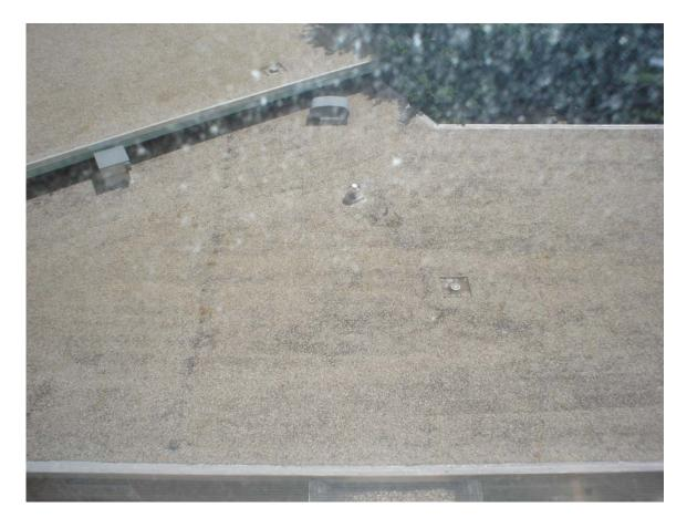
HA #43 – Assumed asbestos-containing roofing products/materials
