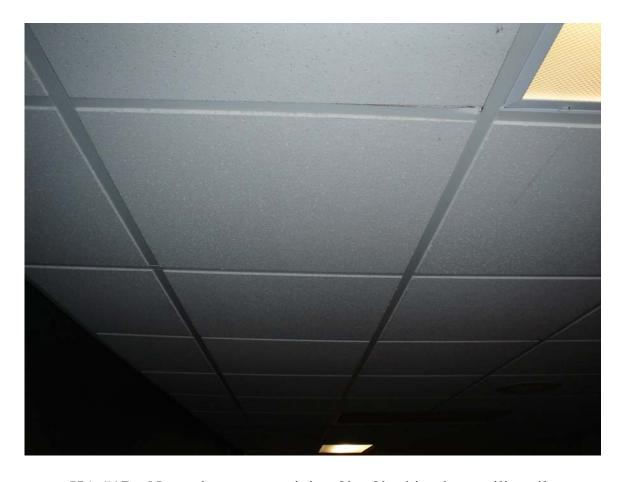
HA #17 – Non asbestos-containing 2' x 2' white drop ceiling tile with pin holes and fissures
