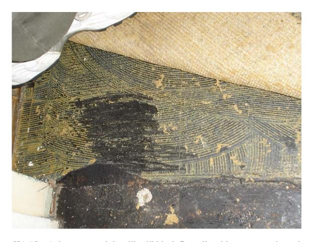
HA #8 – Asbestos-containing 9" x 9" black floor tile with cream streaks and associated non asbestos-containing mastic
