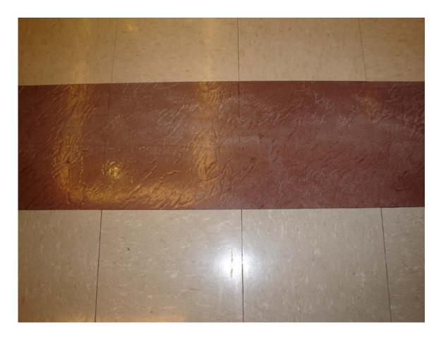
HA #28 – Asbestos-containing 12" x 12" maroon floor tile and associated mastic
