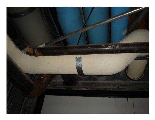
HA #3 – Non asbestos-containing canvas wrap on fiberglass pipe straight insulation
