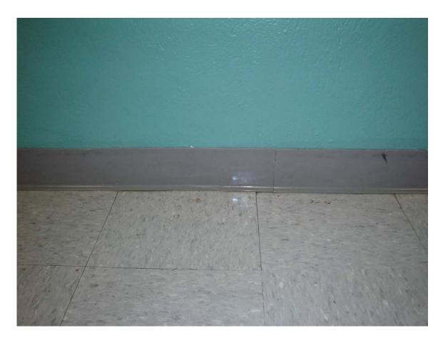
HA #21 – Non asbestos-containing 4" gray cove molding and associated mastic
