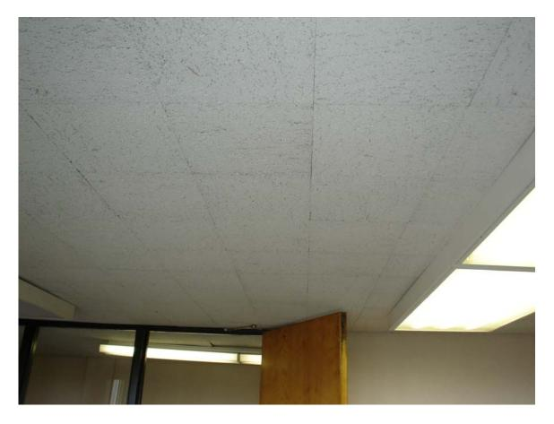
HA #14 – Non asbestos-containing 12" x 12" white ceiling tile with fissures and associated glue pods
