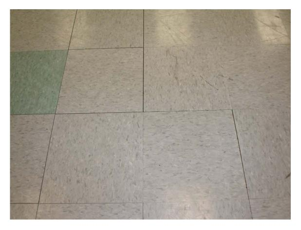
HA #20 – Non asbestos-containing 12" x 12" light gray floor tile with marble pattern and associated mastic
