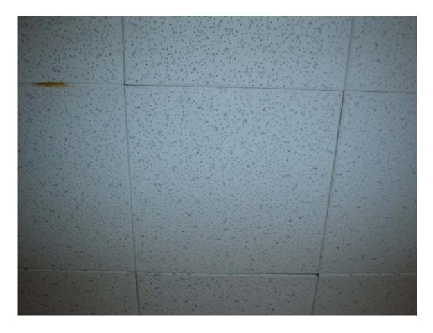
HA #19 – Non asbestos-containing 12" x 12" white ceiling tile with pin holes and fissures and associated glue pods
