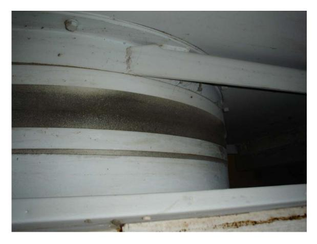
HA #7 – Non asbestos-containing ventilation duct expansion cloth
