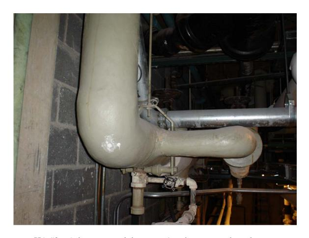
HA #2 – Asbestos-containing steam/condensate supply and return pipe joint and hanger insulation
