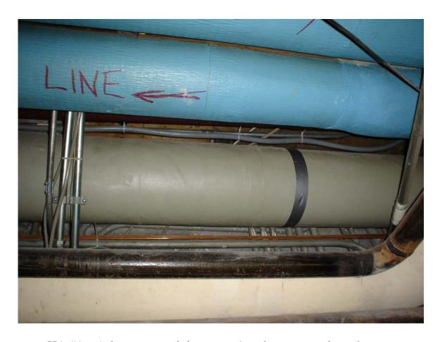
HA #1 – Asbestos-containing steam/condensate supply and return pipe straight insulation
