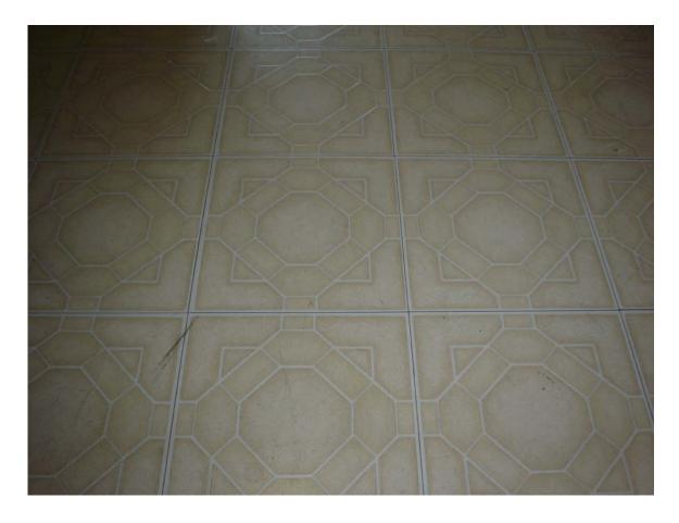
HA #39 – Non asbestos-containing 12" x 12" tan floor tile and associated asbestos-containing mastic
