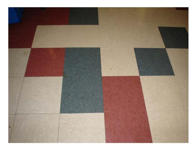
HA #29 – Non asbestos-containing 12" x 12" tan floor tile with marble pattern and associated asbestos-containing mastic
