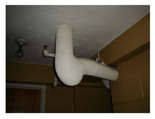
HA #18 – Asbestos-containing drain pipe joint and hanger insulation
