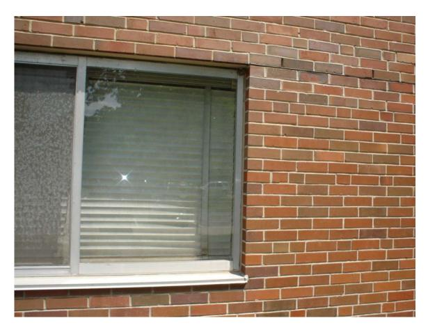
HA #25 – Assumed asbestos-containing window and door frame caulk compound
