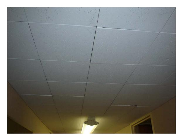
HA #11 – Non asbestos-containing 12" x 12" white ceiling tile with pin holes and associated glue pods
