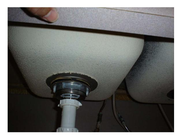
HA #35 – Non asbestos-containing white sink undercoating
