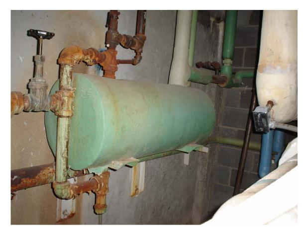
HA #5 – Asbestos-containing hot water holding tank insulation
