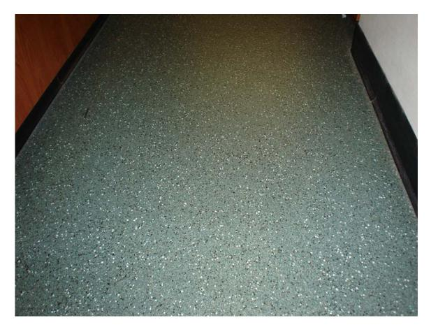
HA #9 - Non asbestos-containing 4" black cove molding and associated mastic
