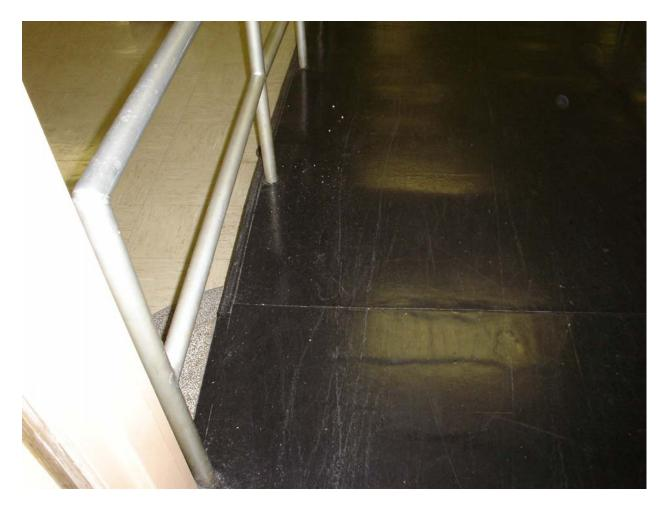
Non-asbestos containing 12" x 12" gray floor tile with cream streaks (painted black) and associated mastic
