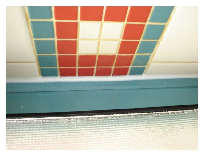
Non-asbestos containing white vinyl floor tile with blue and white chips and associated mastic
