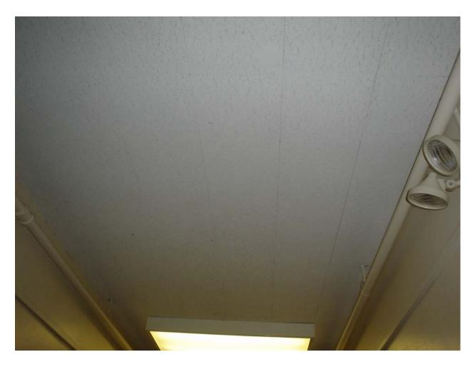
Non-asbestos containing 12" x 12" white ceiling tile with fissures and associated glue pods
