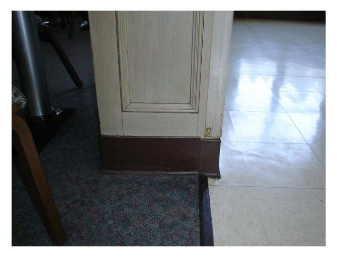
Non-asbestos containing 6" brown cove molding and associated mastic
