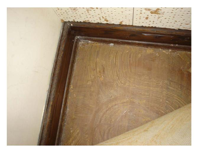
Non-asbestos containing brown floor covering and associated mastic
