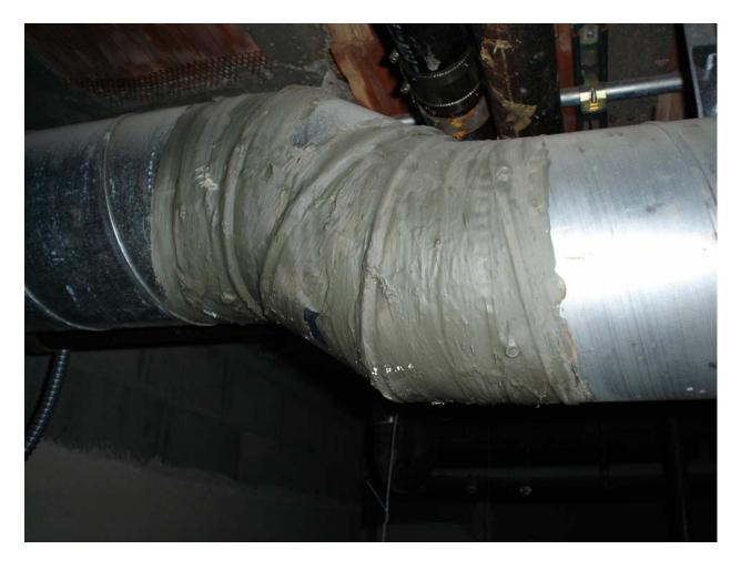
Non-asbestos containing gray duct caulk compound
