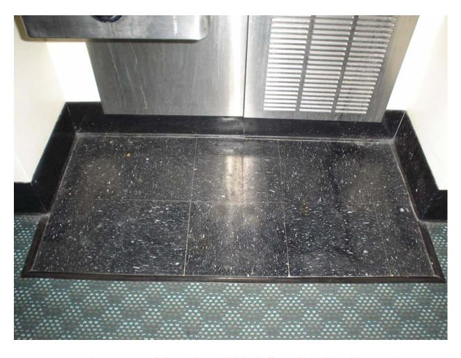
Non-asbestos containing12" x 12" black floor tile with white specks and associated mastic
