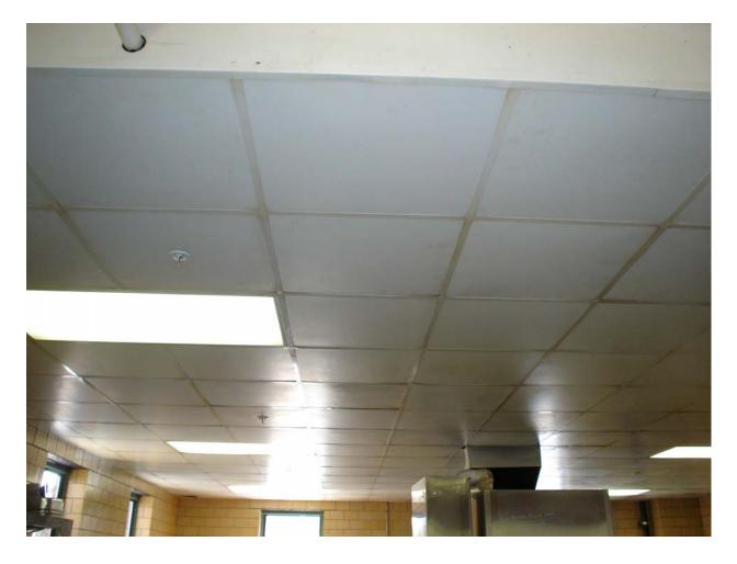
Non-asbestos containing white lay-in ceiling tile with pin holes
