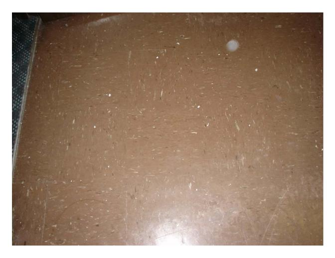
Asbestos-containing 12" x 12" chocolate brown floor tile with cream streaks and associated mastic
