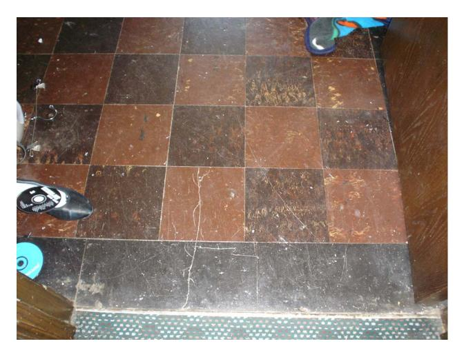
Asbestos-containing 9" x 9" brown floor tile with cream and rust streaks and associated mastic
