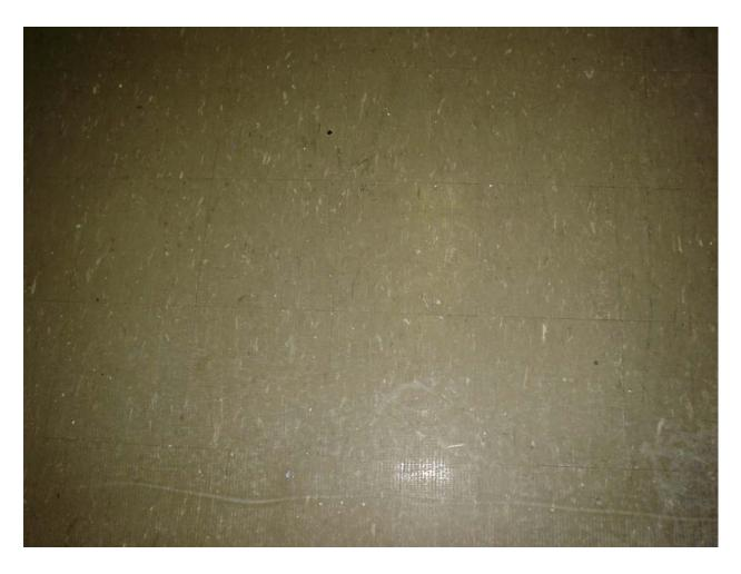
Asbestos-containing 9" x 9" army green floor tile with cream streaks (mastic is non-asbestos containing)
