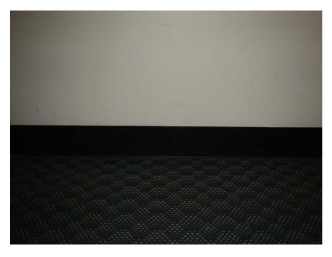
Non-asbestos containing 6" black cove molding and associated mastic
