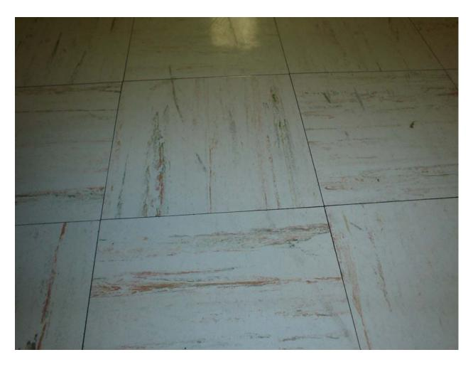
Asbestos-containing 9" x 9" cream floor tile with pink and green streaks (mastic is non-asbestos containing)
