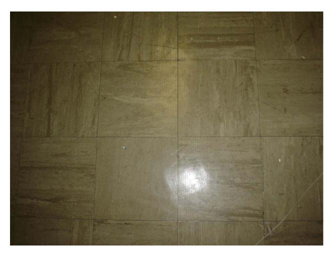
Asbestos-containing 9" x 9" beige floor tile with swirls (mastic is non-asbestos containing)
