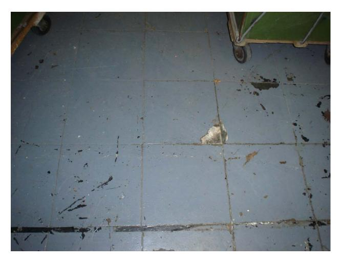
Asbestos-containing 12" x 12" brown floor tile and associated mastic (painted gray in Laundry #7)
