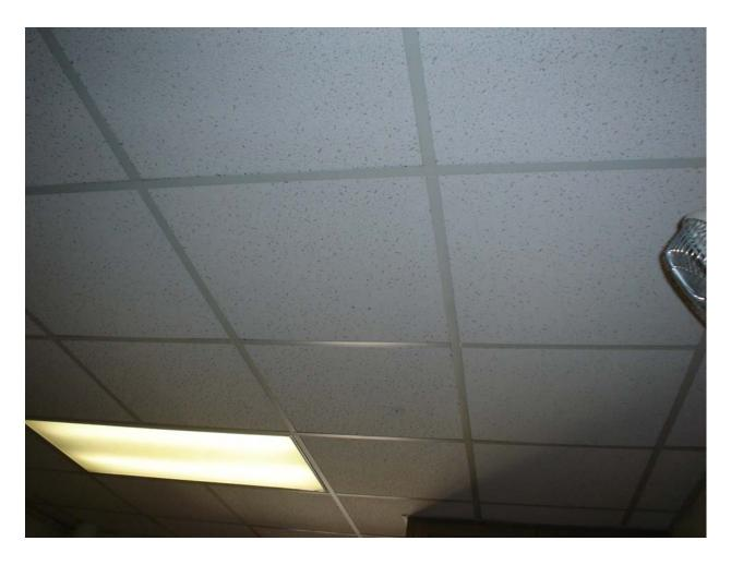
Non-asbestos containing 2' x 2' white lay-in ceiling tile with fissures
