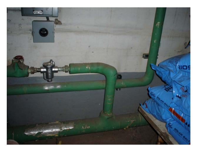
Asbestos-containing steam/condensate supply & return pipe straight insulation
