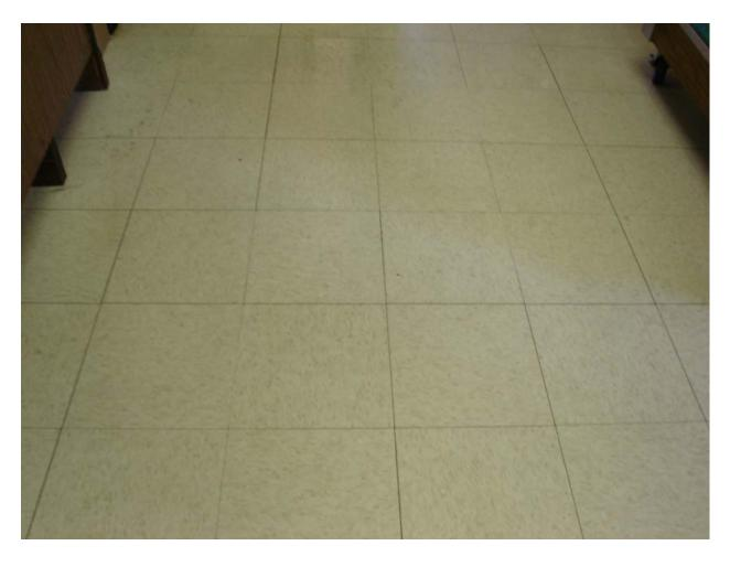
Non-asbestos containing 12" x 12" cream marble pattern floor tile and associated mastic
