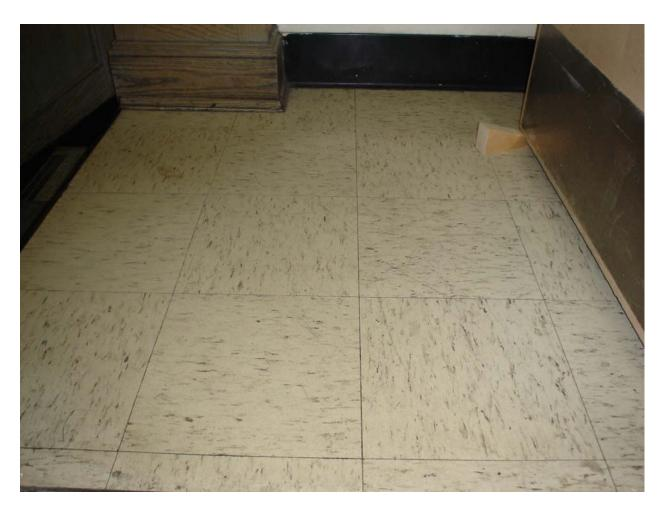
Non-asbestos containing 12" x 12" cream floor tile with tan and rust streaks (mastic is asbestos-containing)
