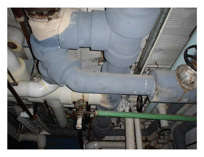
Asbestos-containing steam/condensate supply & return pipe joint insulation
