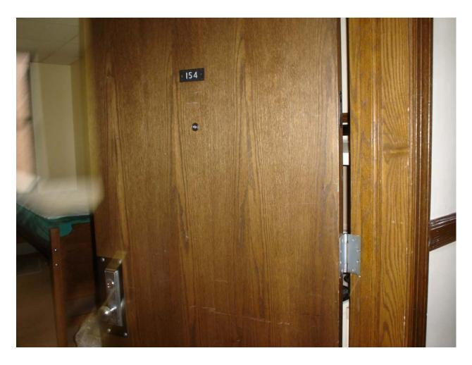
Assumed asbestos-containing fire door and frame
