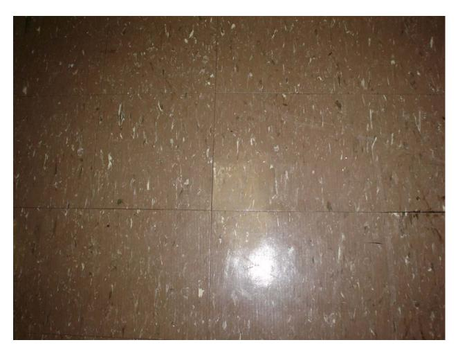
Asbestos-containing 9" x 9" chocolate brown floor tile with cream streaks (mastic is non-asbestos containing)
