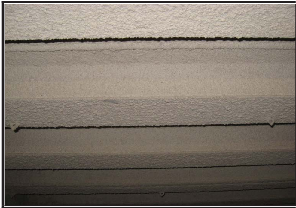
HA-20 Spray-on fire proofing on structural steel and deck
