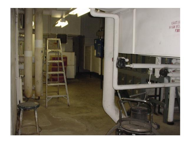
Mechanical Room 306 – thermal system insulation and duct wrap
