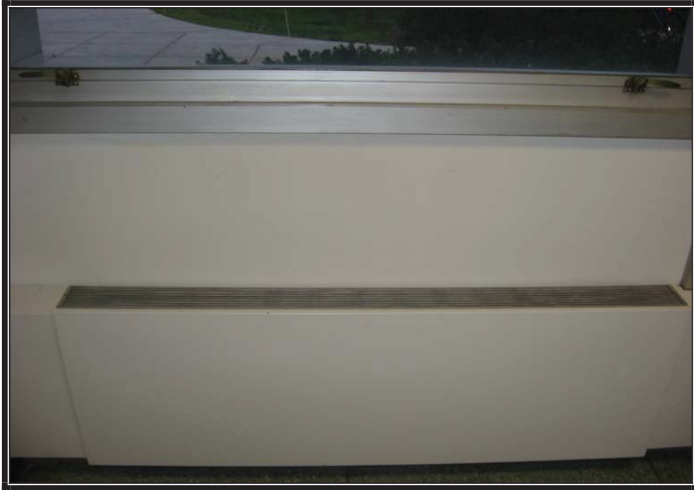
HA43 – Transite Wall Panels
