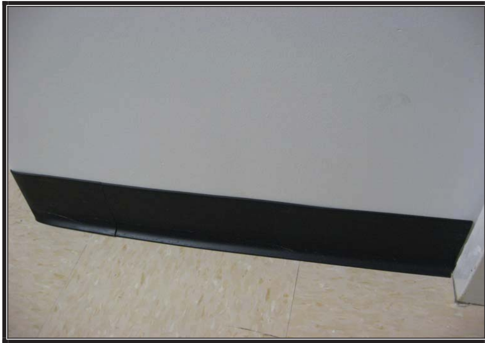
HA33 – Black Covebase (1985 Addition)
