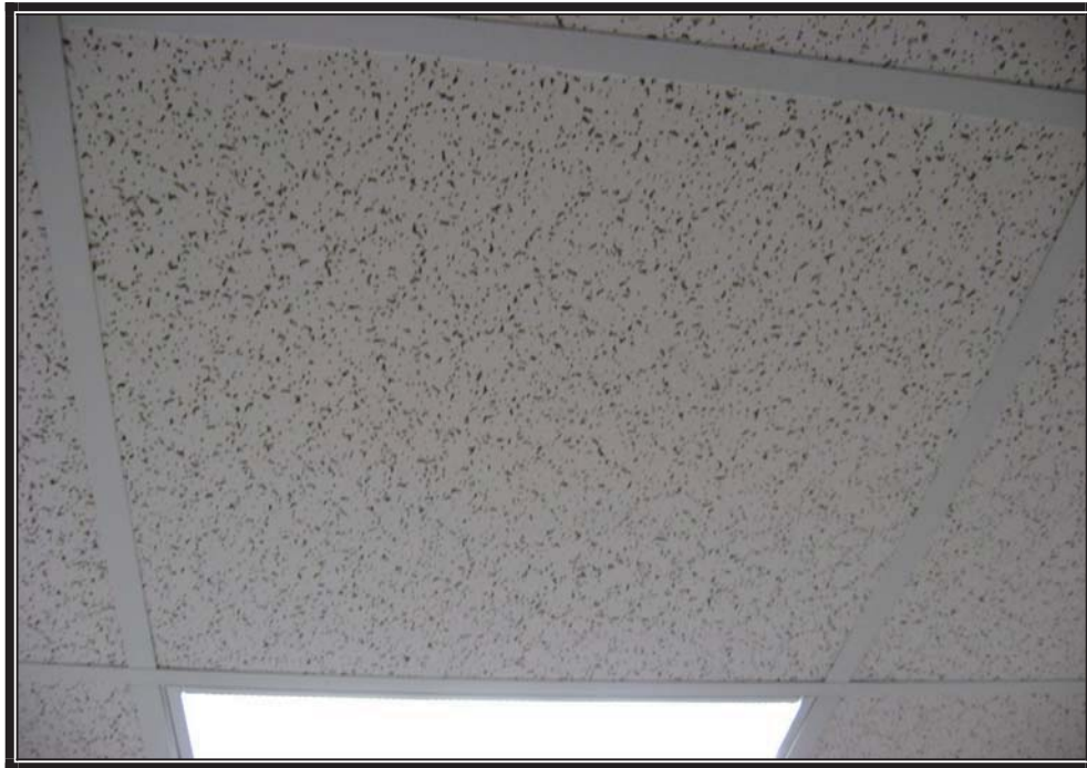
HA37 – 2' x 2' Suspended Ceiling (1985 Addition)
