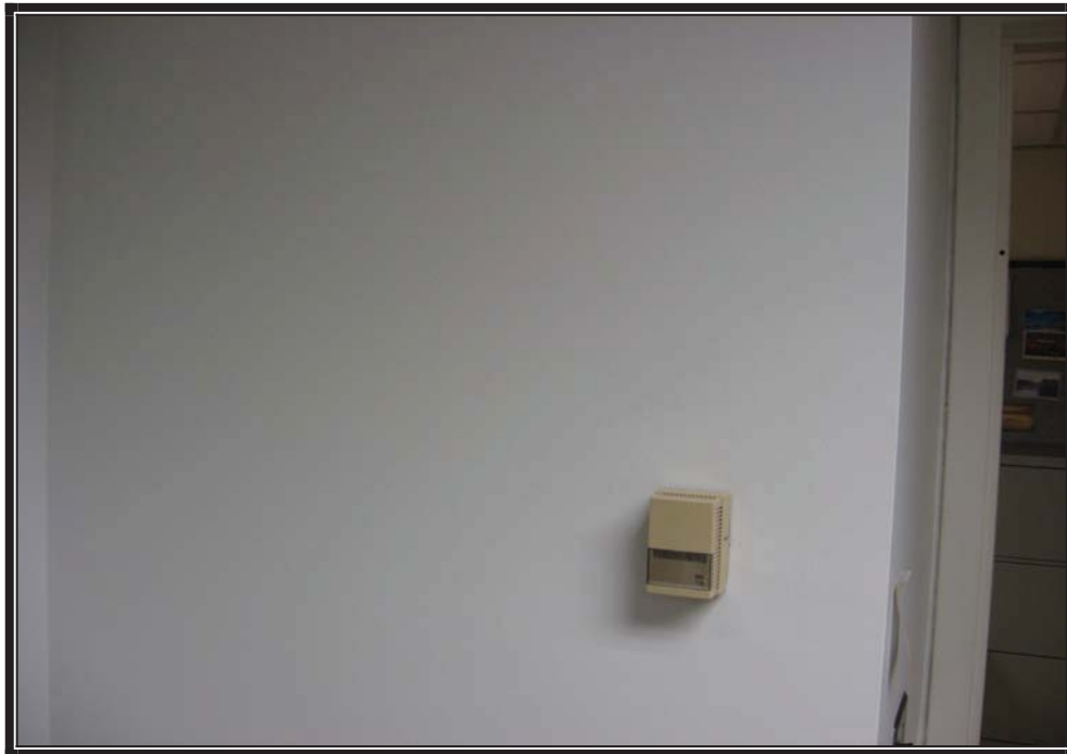
HA34 – Drywall (1985 Addition)
