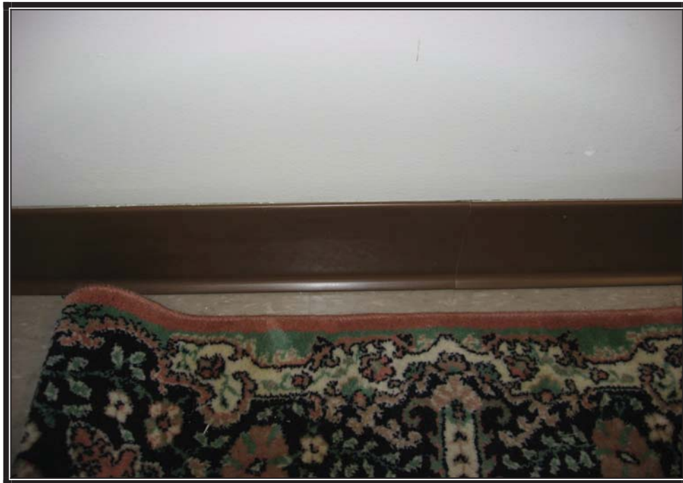
HA47 – Reddish Brown Covebase (1985 Addition)
