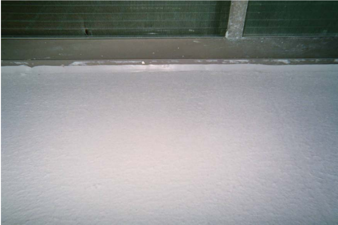
Photo 19 – Assumed asbestos-containing caulk compound
