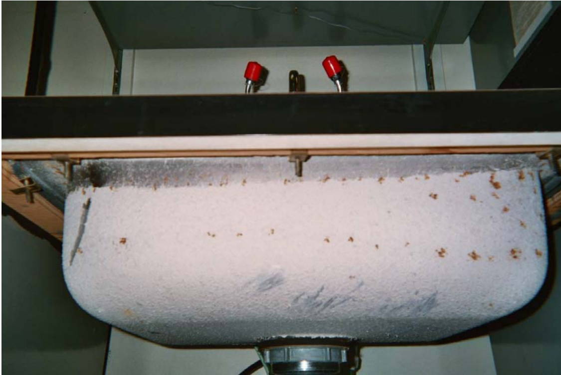
Photo 10 – Non asbestos-containing pink sink undercoating
