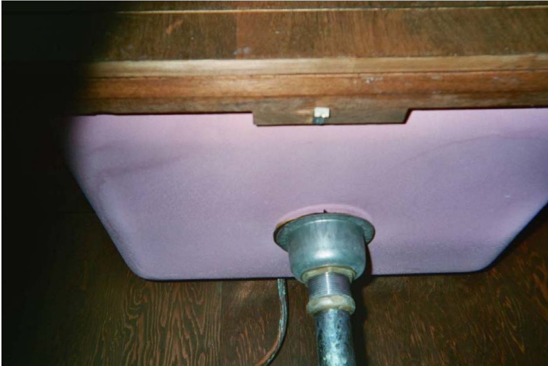
Photo 13 – Non asbestos-containing pink sink undercoating
