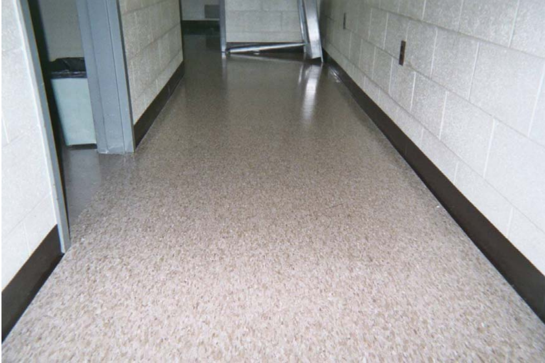
Photo 16 – Asbestos-containing 12” x 12” tan marble floor tile
