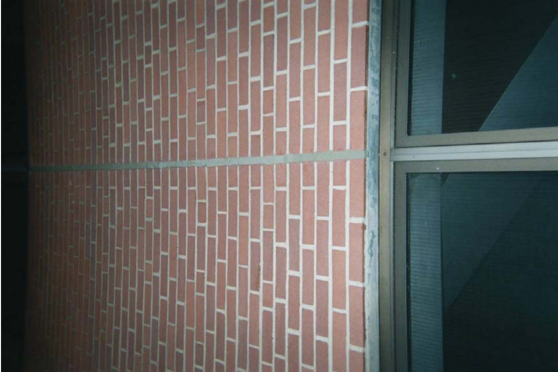
Photo 20 – Assumed asbestos-containing caulk compound
