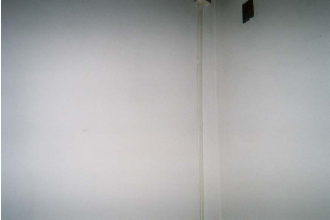
Photo 9 – Non asbestos-containing plaster
