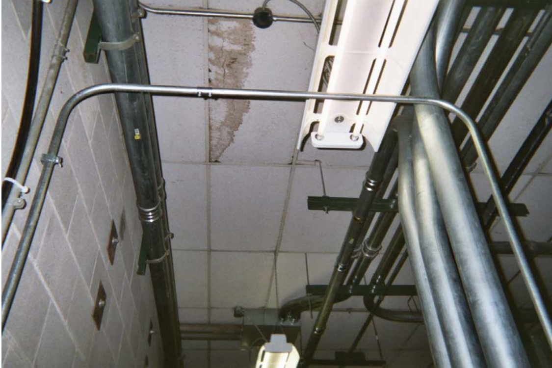
Photo 15 – Non asbestos-containing 2' x 4' white lay-in ceiling tile with pin holes and fissures
