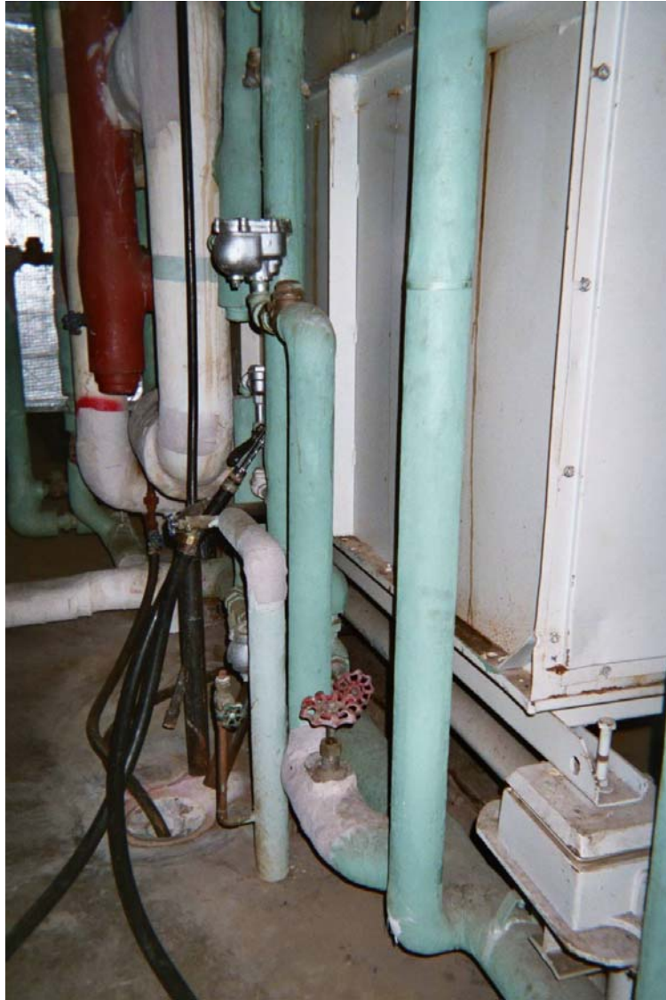
Photo 1 – Non asbestos-containing domestic water pipe straight insulation
