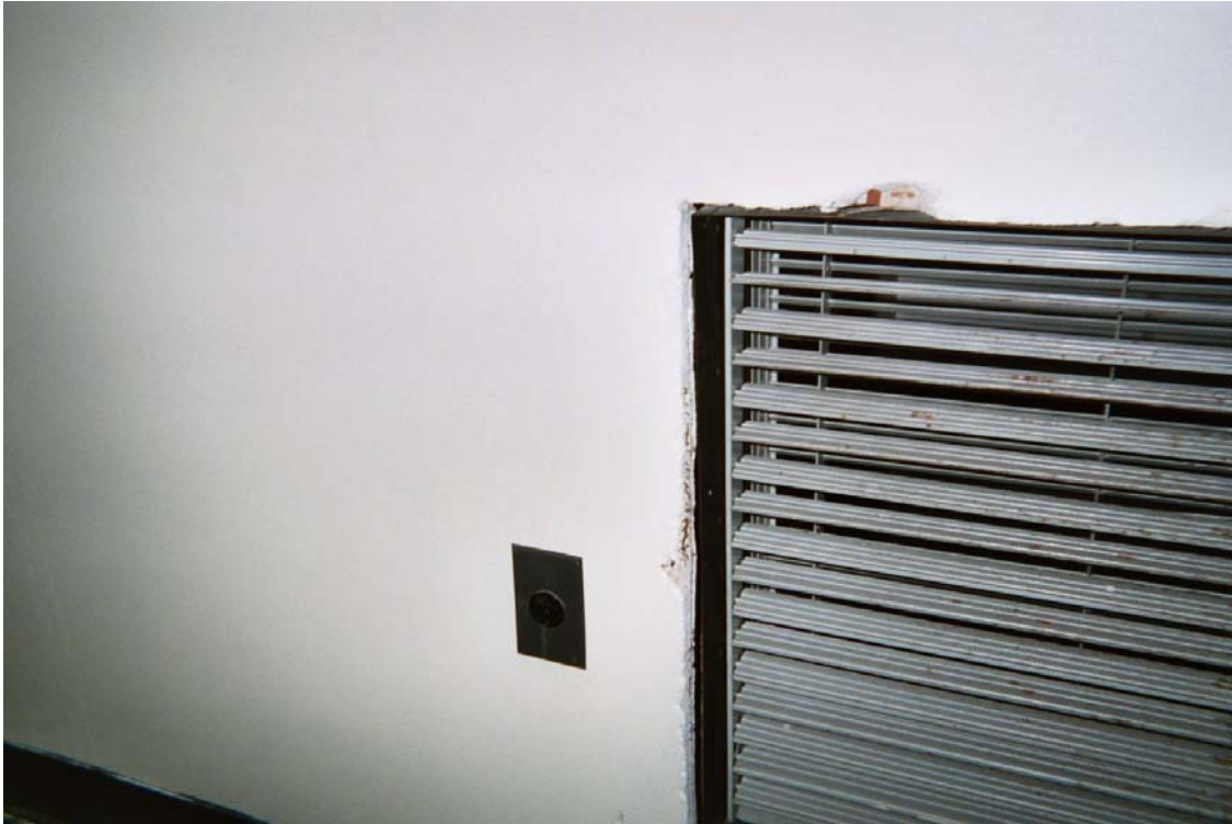
Photo 12 – Non asbestos-containing plaster
