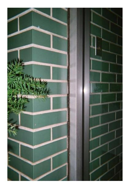
Photo 6 - Assumed asbestos-containing black building caulk compound
