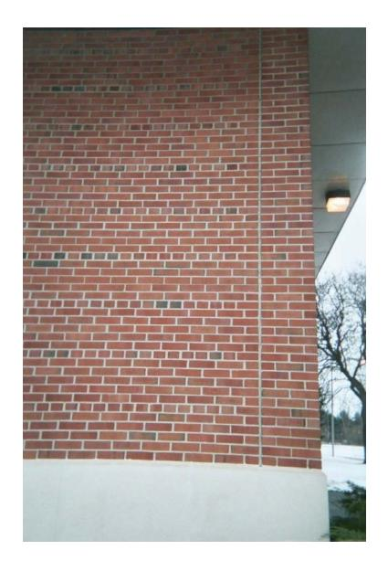
Photo 1 - Assumed asbestos-containing gray building caulk compound
