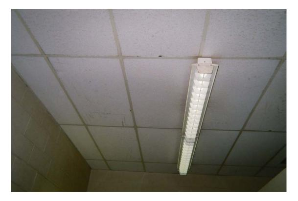
Photo 11 – Non asbestos-containing 2' x 4' white lay-in ceiling tile with pin holes and fissures
