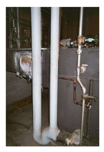
Photo 21 - Non asbestos-containing domestic water pipe straight insulation
