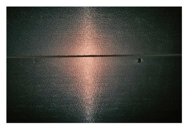
Photo 16 – Non asbestos-containing gray refrigeration caulk compound
