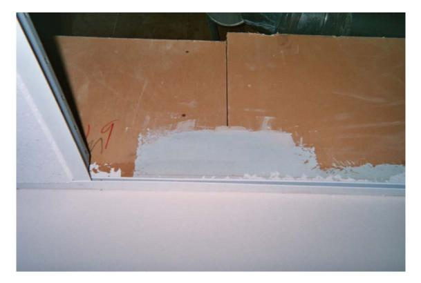
Photo 12 - Asbestos-containing drywall joint compound
