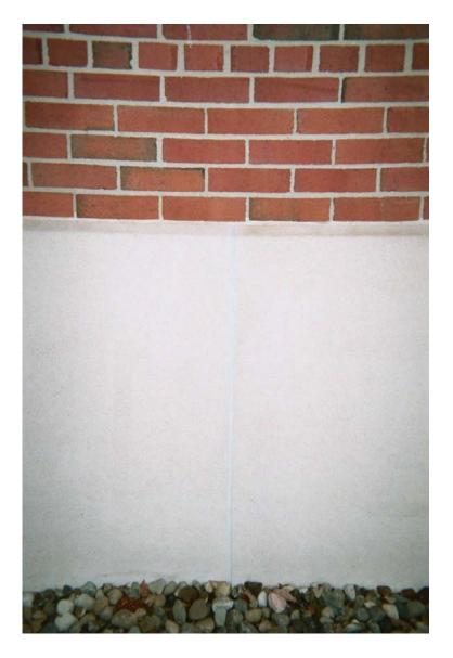
Photo 3 – Assumed asbestos-containing gray building caulk compound
