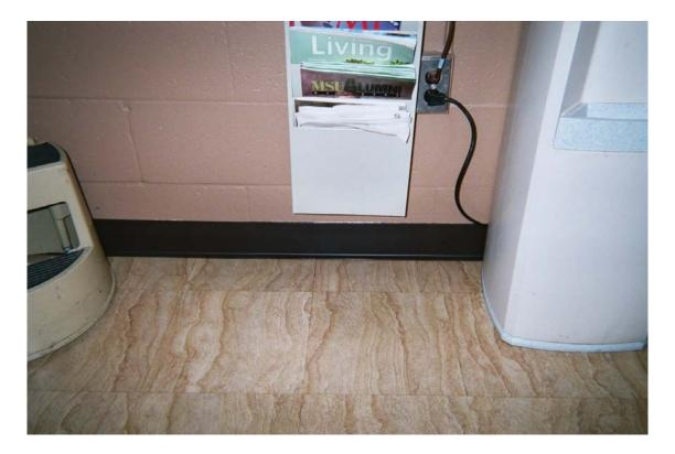
Photo 9 – Non asbestos-containing 4" black cove molding and associated mastic
