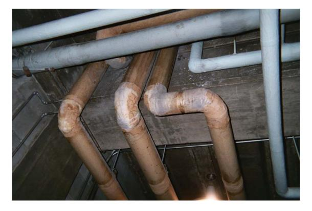
Photo 20 - Asbestos-containing domestic water pipe joint insulation
