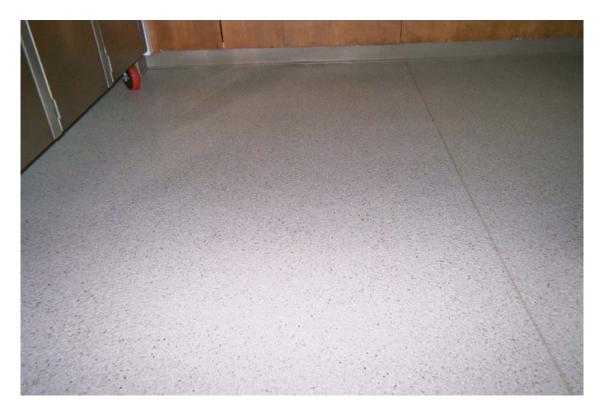
Photo 8 – Non asbestos-containing cream and vinyl flooring with tan specks and associated mastic
