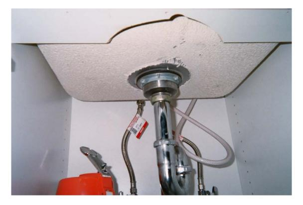
Photo 15 – Non asbestos-containing cream sink undercoating
