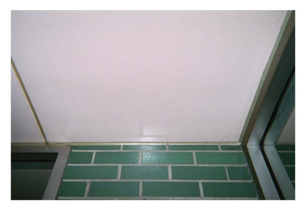
Photo 7 – Assumed asbestos-containing green building caulk compound
