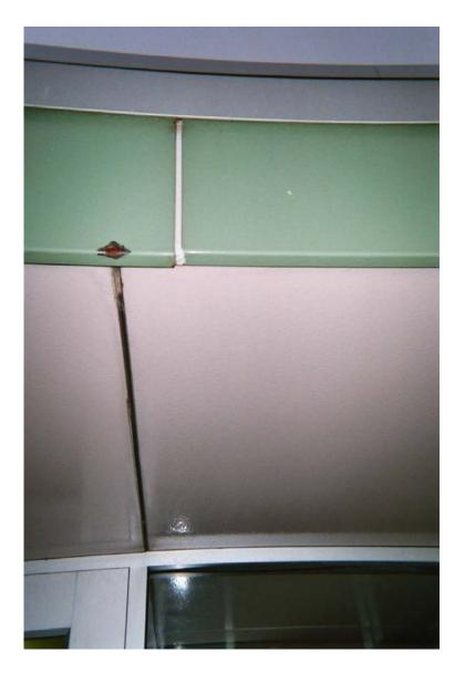
Photo 5 – Assumed asbestos-containing white and black exterior building caulk compound
