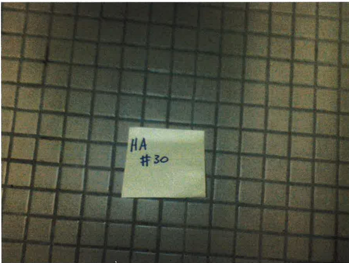
HA #30 – Non asbestos-containing 1/2" x 1/2" solid gray ceramic floor tile bedding compound and grout
