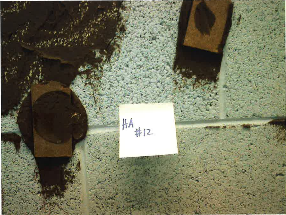
HA #12 – Non asbestos-containing brown glue pods
