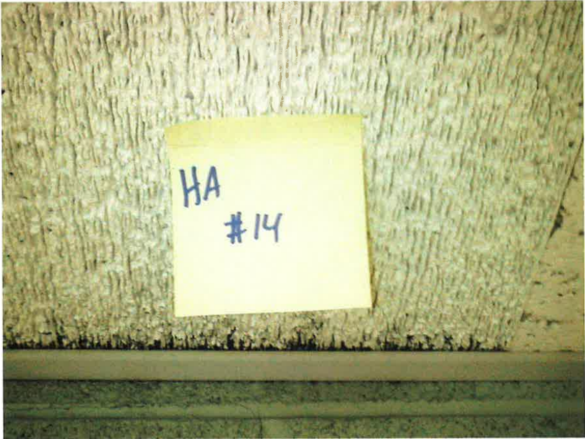
HA #14 – Non asbestos-containing 1' x 1' white spline ceiling tile with lines
