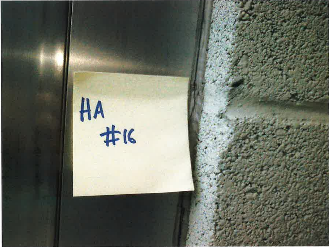
HA #16 – Non asbestos-containing interior silver window caulk compound
