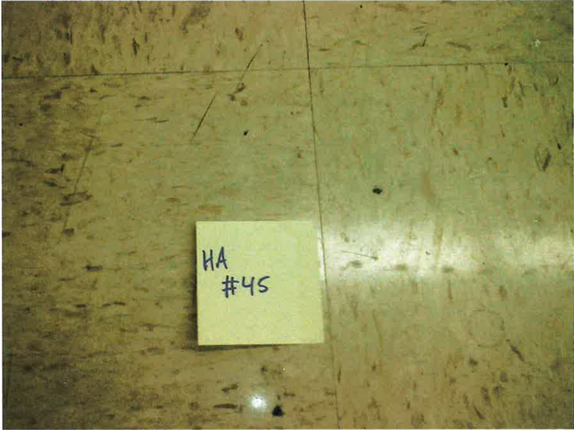
HA #45 – Non asbestos-containing 12" x 12" light brown floor tile with brown streaks and associated mastic
