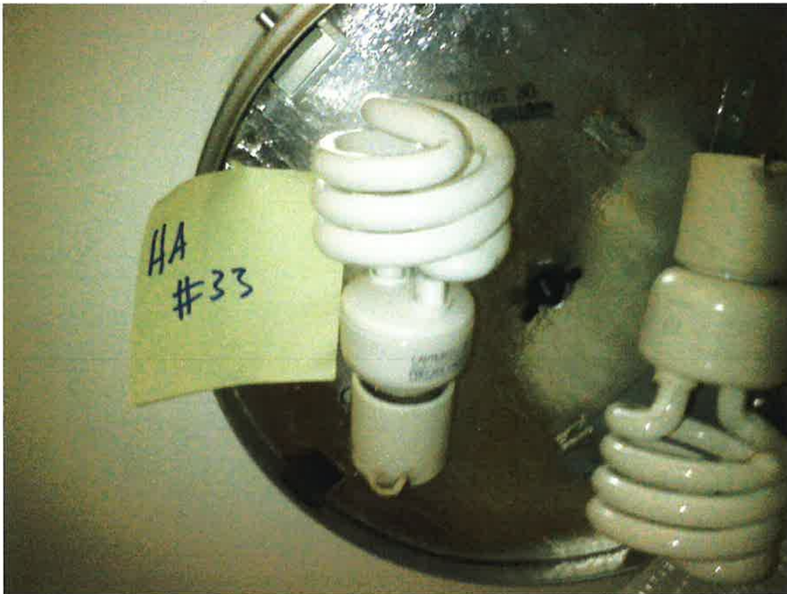
HA #33 – Asbestos-containing light reflector paper
