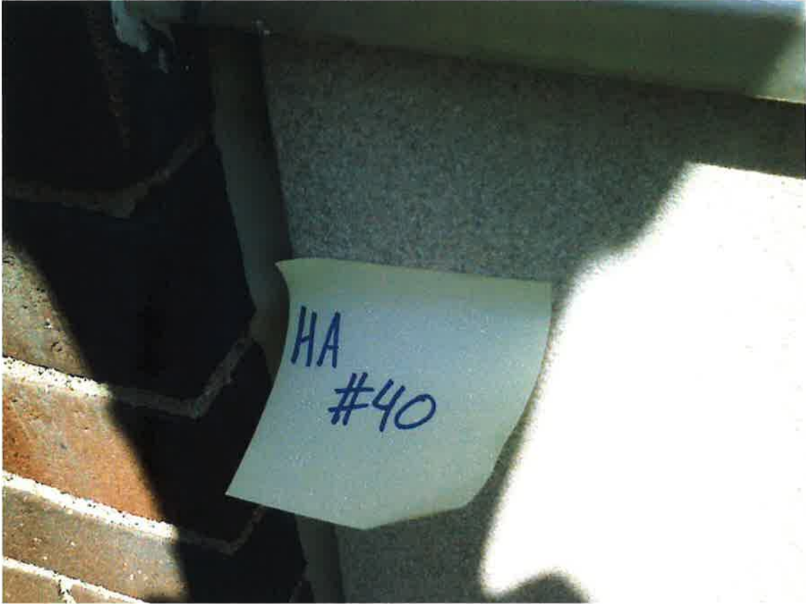
HA #40 – Non asbestos-containing exterior gray building caulk compound
