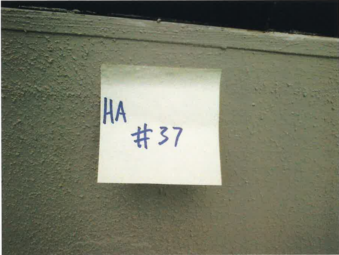
HA #37 – Non asbestos-containing exterior textured plaster
