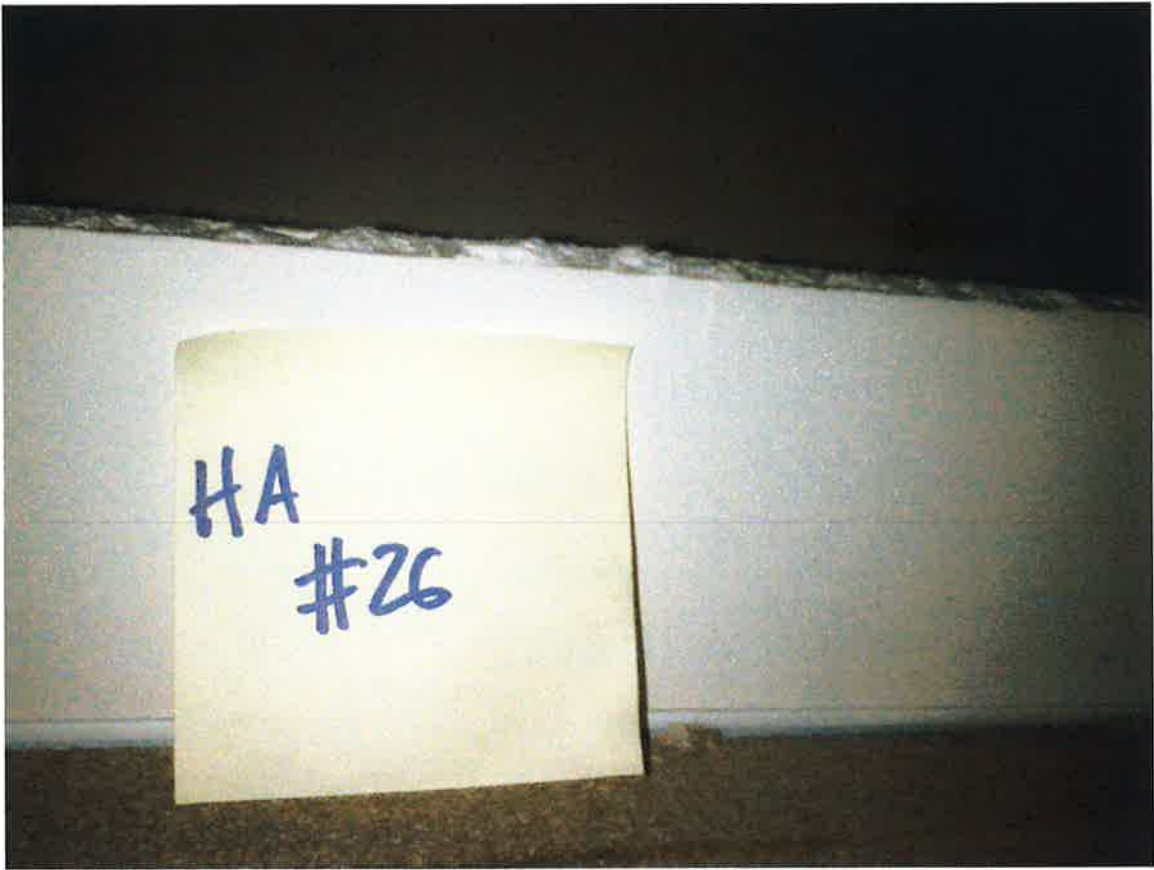
HA #26 – Non asbestos-containing drywall
