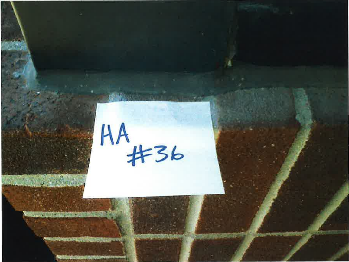
HA #36 – Non asbestos-containing exterior brown window, door and building caulk compound
