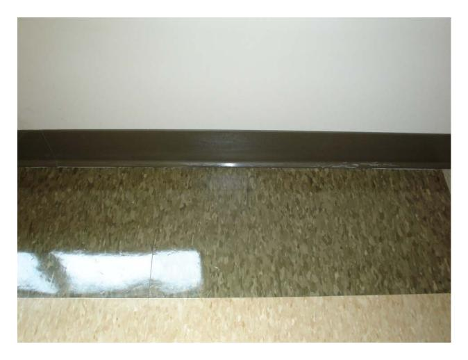
Non-asbestos containing 4" army green cove molding and associated mastic
