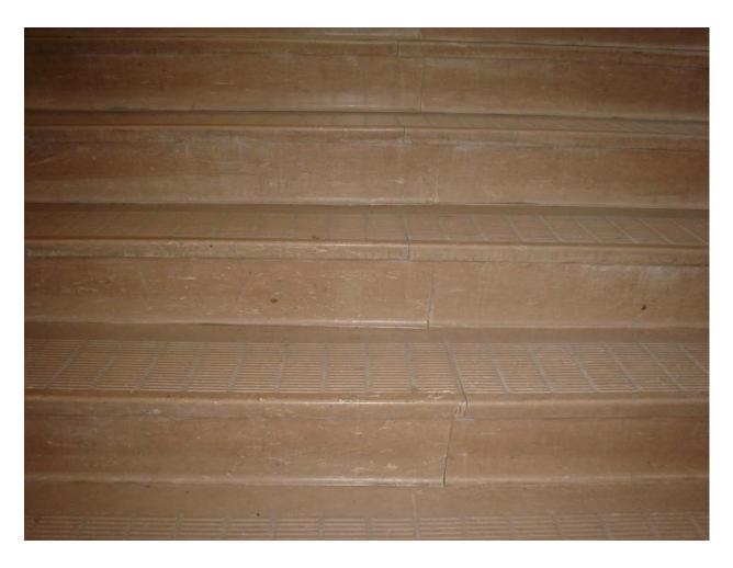
Non-asbestos containing tan stair tread with cream and brown streaks and associated mastic
