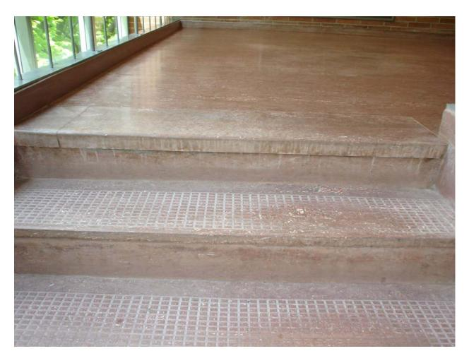
Asbestos-containing vinyl stair tread with white streaks (mastic is non-asbestos containing)
