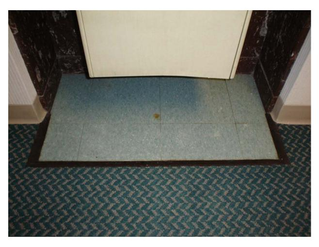
Non-asbestos containing 12" x 12" green marble pattern floor tile and associated mastic
