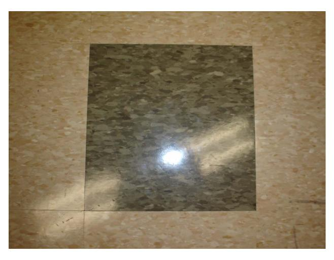
Non-asbestos containing 12" x 12" army green marble pattern floor tile and associated mastic
