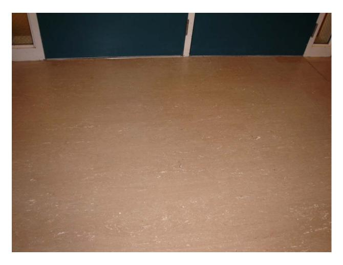
Non-asbestos containing 12" x 12" tan linoleum squares with cream and brown streaks and associated mastic
