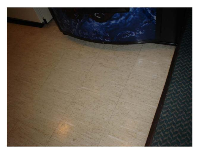
Non-asbestos containing 12" x 12" beige floor tile with cream and green streaks and associated mastic
