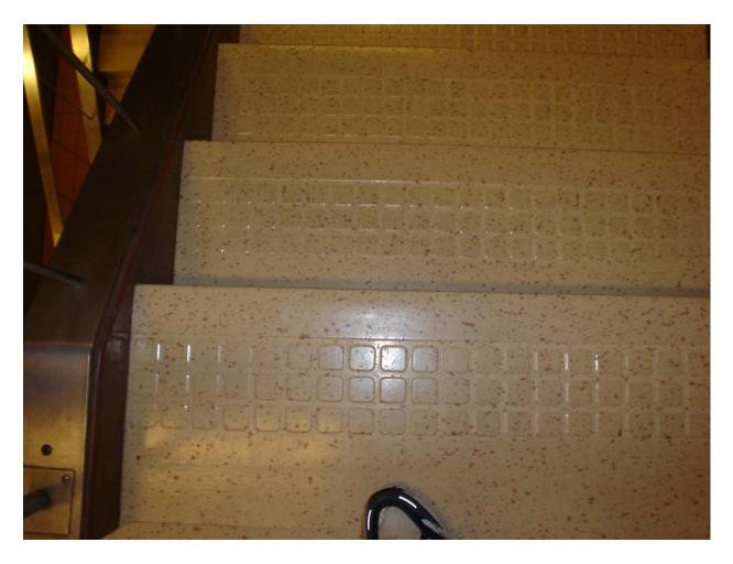
Non-asbestos containing tan stair tread with multicolored specks and associated mastic
