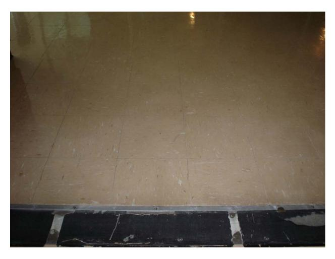
Non-asbestos containing 12" x 12" tan floor tile with white and rust streaks (mastic is asbestos-containing)
