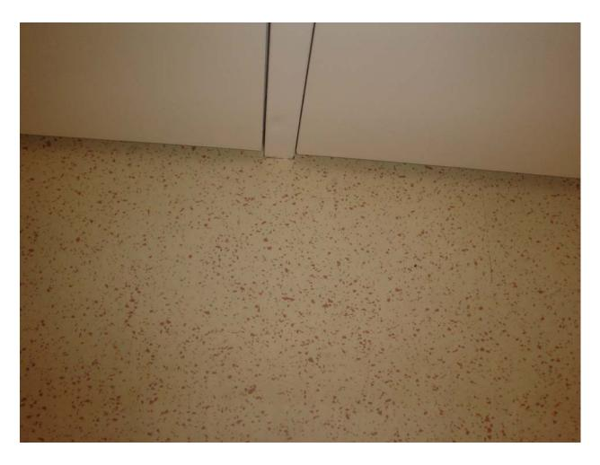
Non-asbestos containing 2' x 2' tan vinyl flooring with multicolored specks and associated mastic
