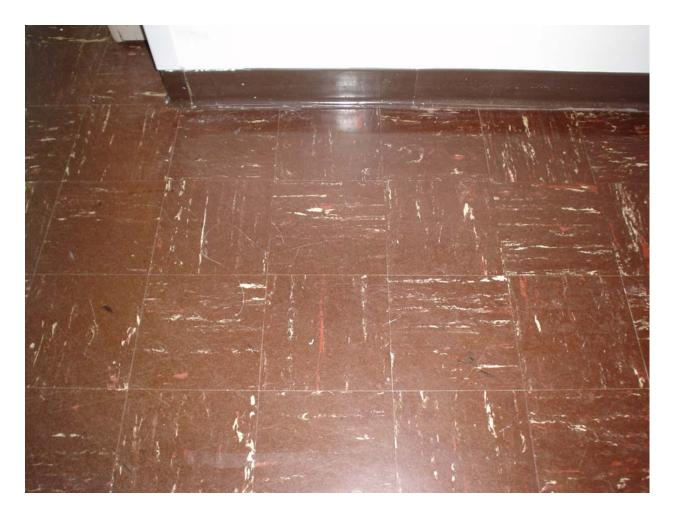
Non-asbestos containing 4" brown cove molding and associated mastic
