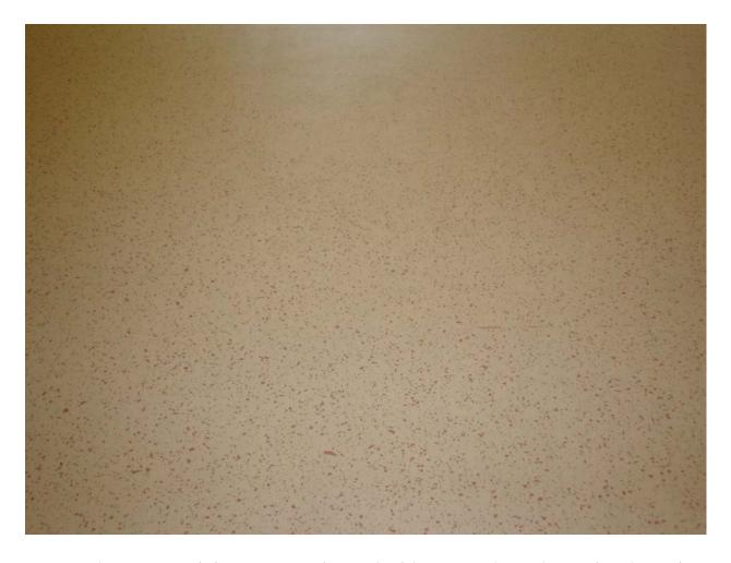
Non-asbestos containing cream stair tread with tan specks and associated mastic
