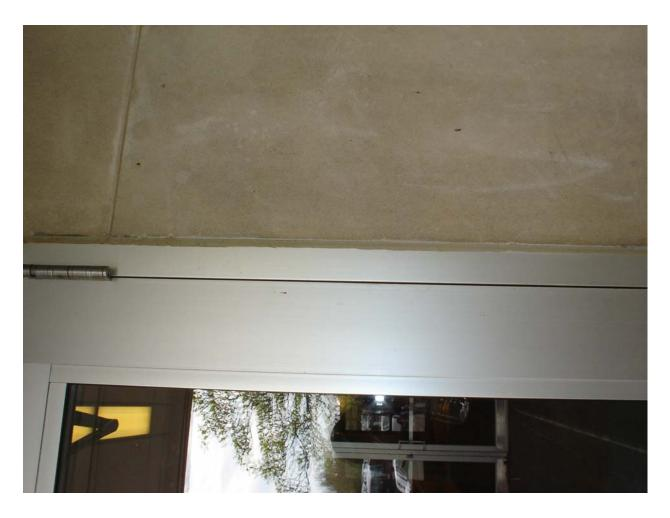
Assumed asbestos-containing window and door frame caulk compound
