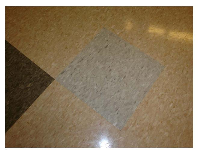
Non-asbestos containing 12" x 12" gray marble pattern floor tile and associated mastic
