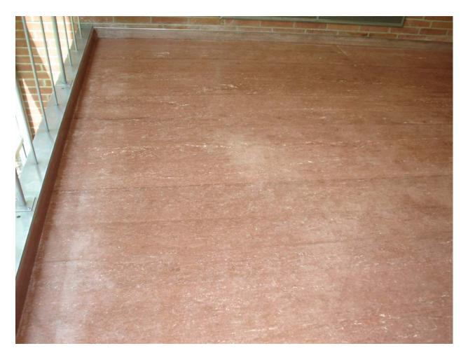
Asbestos-containing red linoleum with white streaks (mastic is non-asbestos containing)
