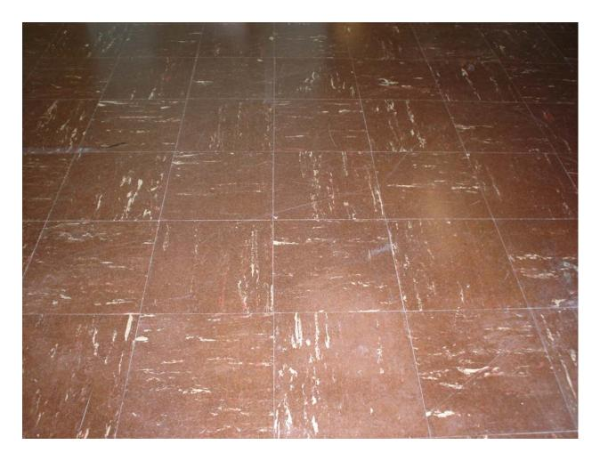
Non-asbestos containing 12" x 12" brown floor tile with cream and green streaks and associated mastic
