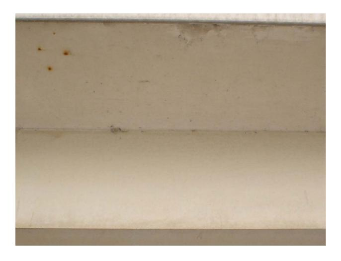
Non-asbestos containing plaster (smooth)
