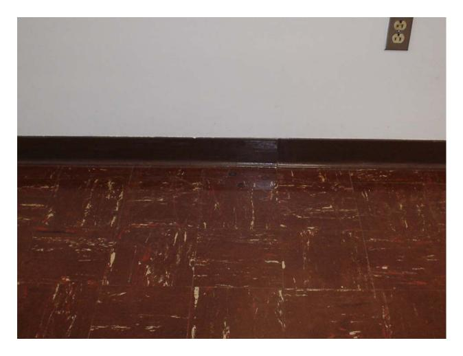
Asbestos-containing 9" x 9" dark brown floor tile with cream and rust streaks and associated mastic
