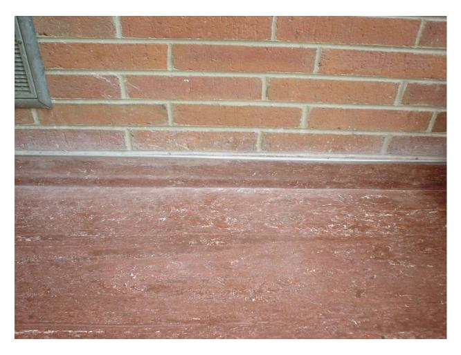
Asbestos-containing 4" red cove molding with white streaks (mastic is non-asbestos containing)
