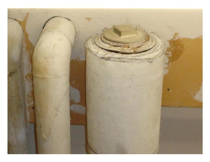
Asbestos-containing drain system pipe straight insulation
