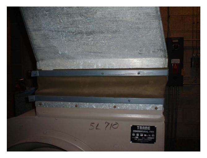
Non-asbestos containing ventilation duct expansion cloth
