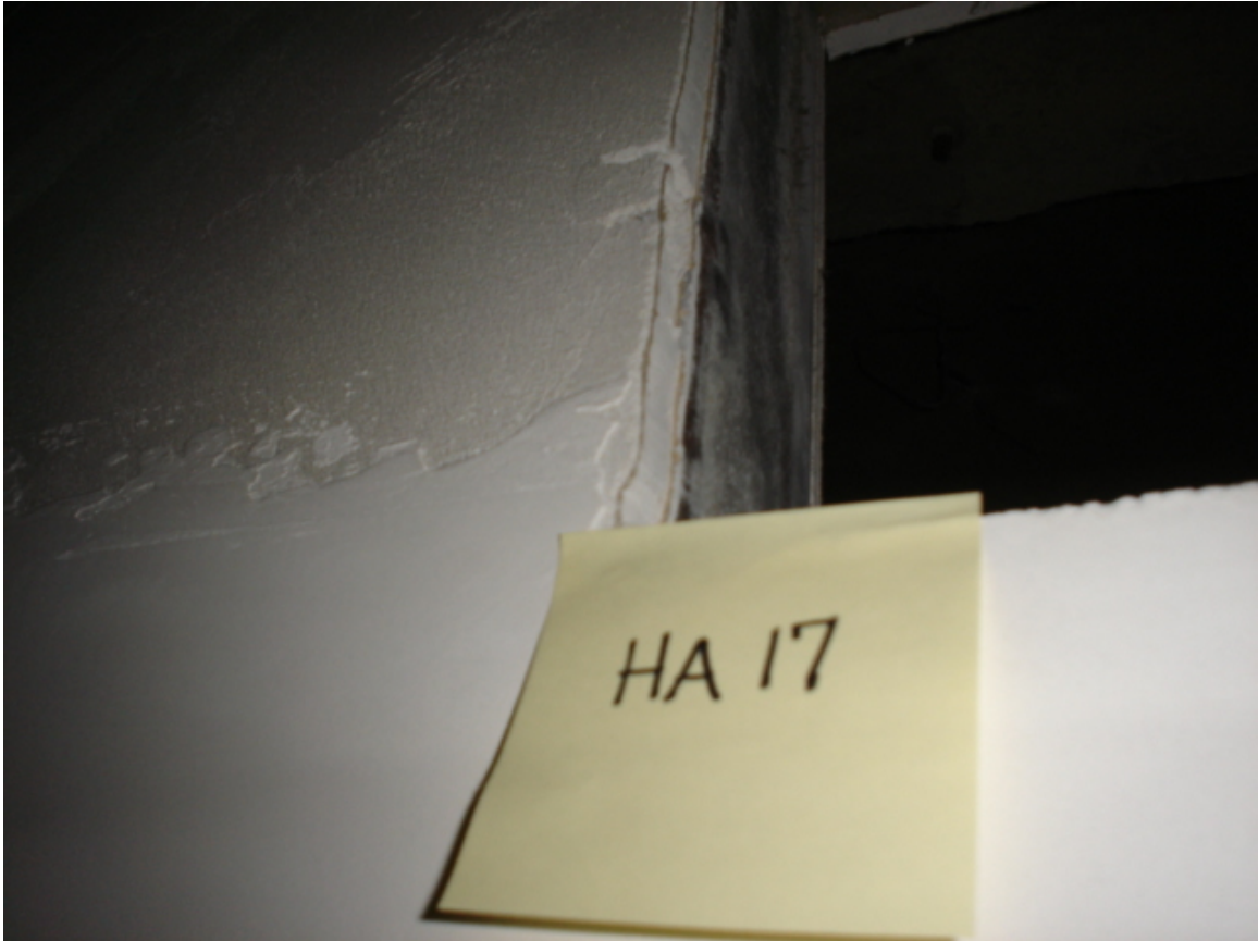
HA #17 – Non asbestos-containing drywall
