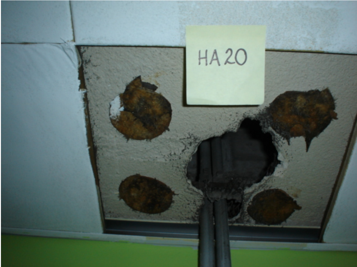
HA #20 – Non asbestos-containing glue pods from 12" x 12" fiberglass ceiling tile
