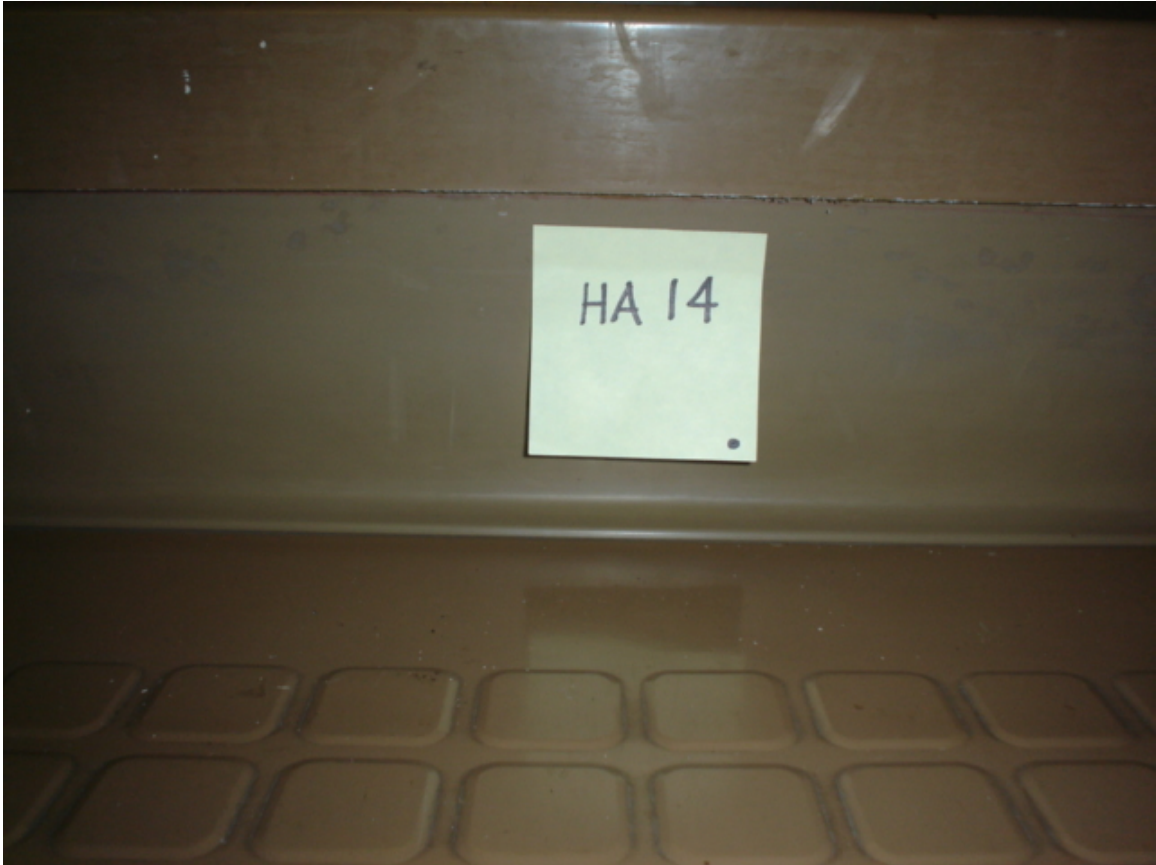
HA #14 – Non asbestos-containing 6" tan cove molding and associated mastic
