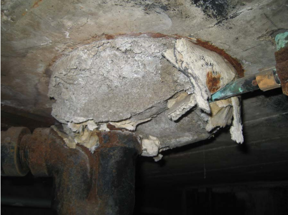
HA #6 – Non-asbestos containing corrugated material
