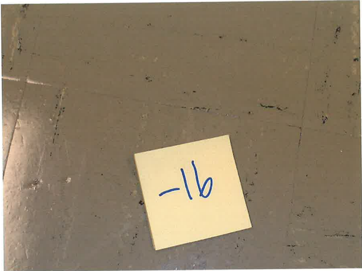
HA #16 – Asbestos containing 9” x 9” gray floor tile with black and cream streaks and non asbestos containing associated mastic
