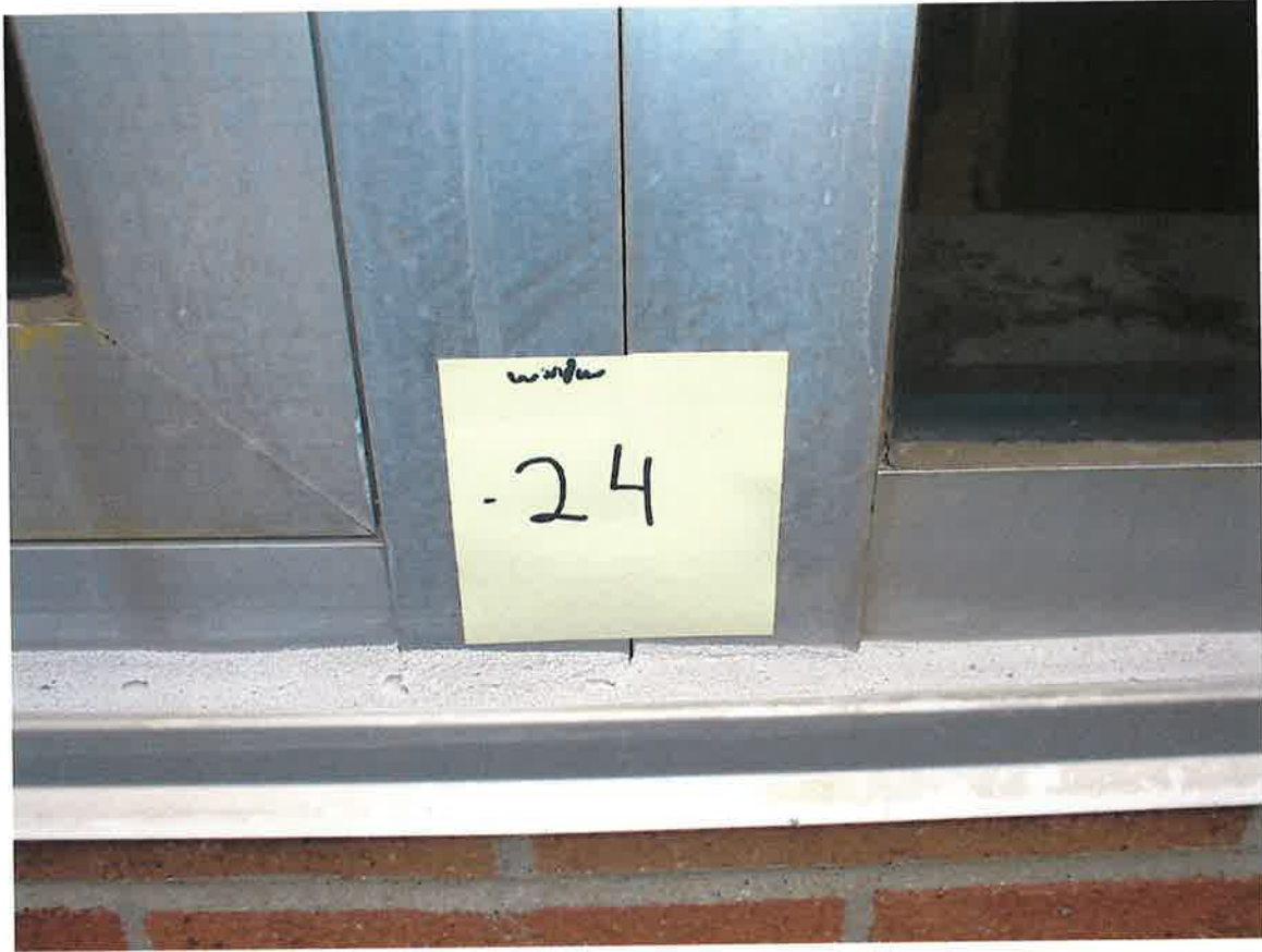
HA #24 – Non asbestos containing window and door frame caulk compound (exterior)
