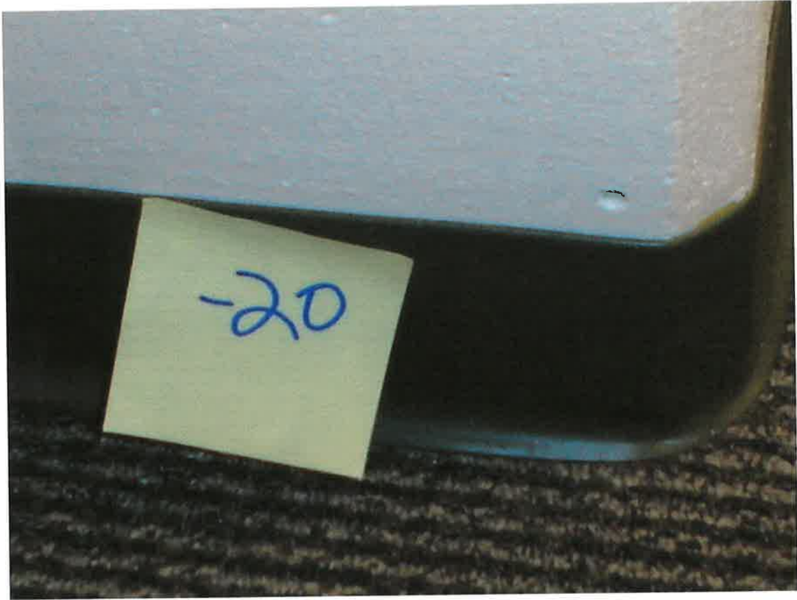
HA #20 – Non asbestos containing 4” olive green cove molding and associated mastic
