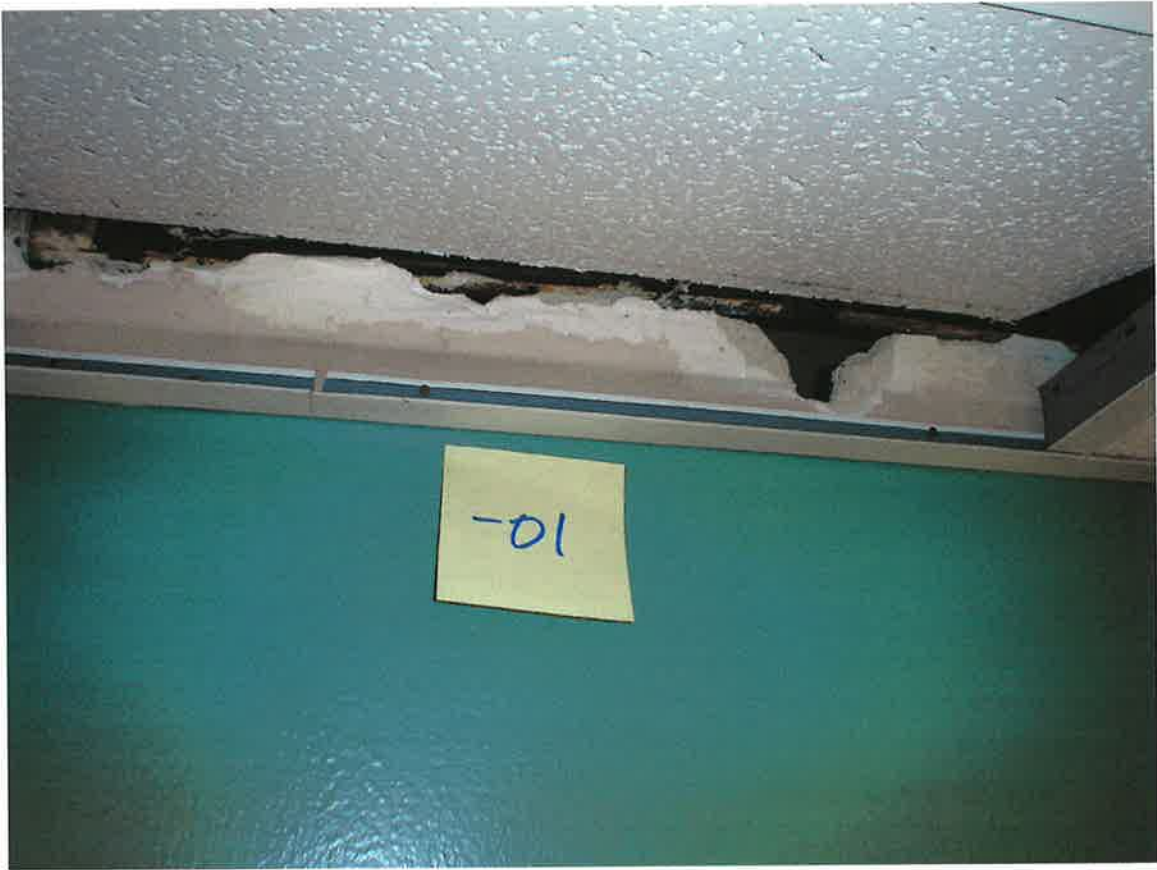
HA #1 – Non asbestos containing smooth plaster over drywall
