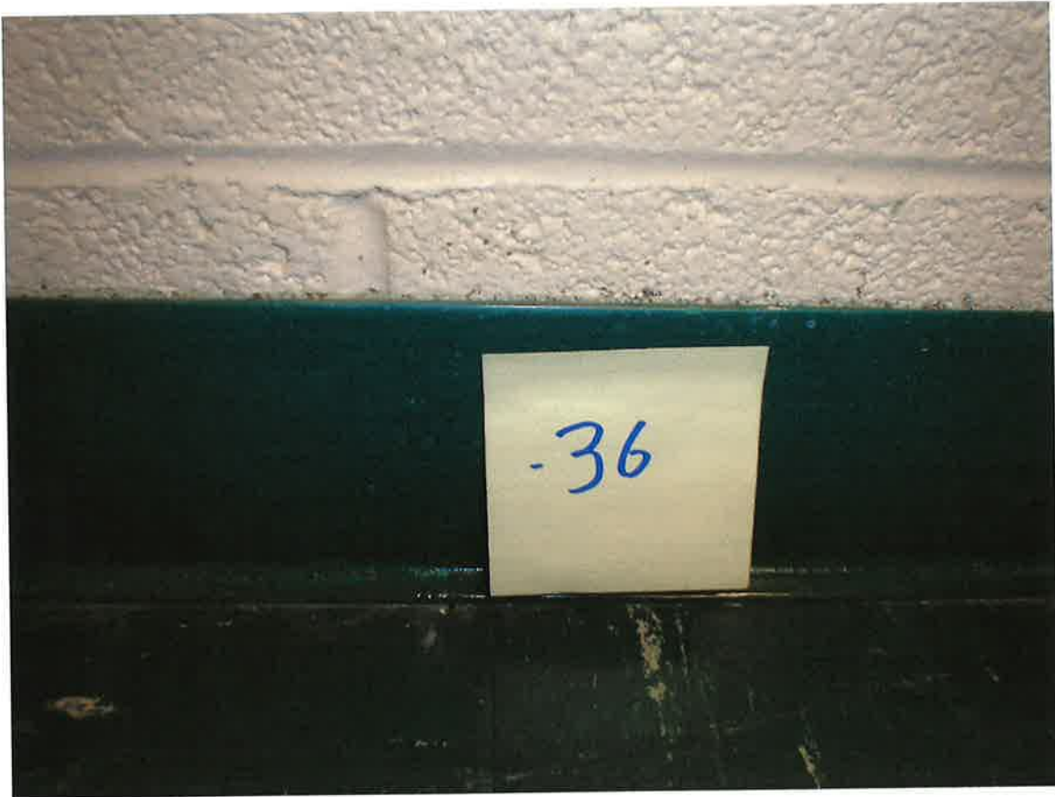
HA #36 – Non asbestos containing 4" green cove molding and associated mastic
