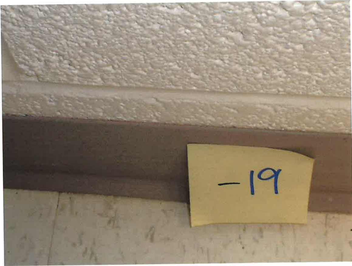
HA #19 – Non asbestos containing 4” gray cove molding and associated mastic
