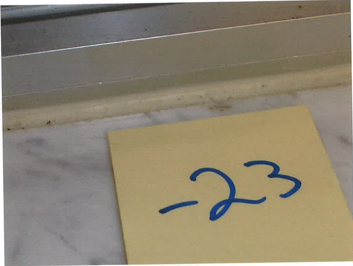
HA #23 – Non asbestos containing window and door frame caulk compound (interior)
