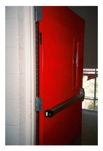
HA #27 – Assumed asbestos-containing fire door and frame
