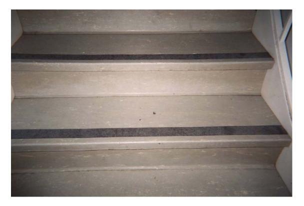
HA #15 – Non asbestos-containing gray stair tread with cream streaks and associated mastic
