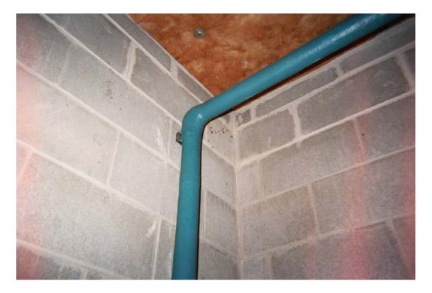
HA #21 – Asbestos-containing domestic water supply pipe joint and hanger insulation
