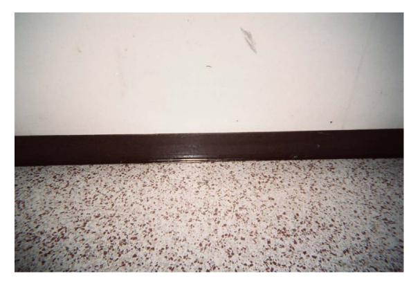
HA #8 – Non asbestos-containing 4" dark brown cove molding and associated mastic
