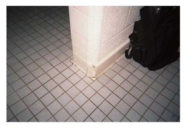
HA #28 – Non asbestos-containing ceramic tile bedding compound
