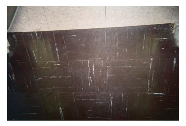
HA #29 – Non asbestos-containing 9" x 9" dark brown floor tile with cream and rust streaks and associated mastic
