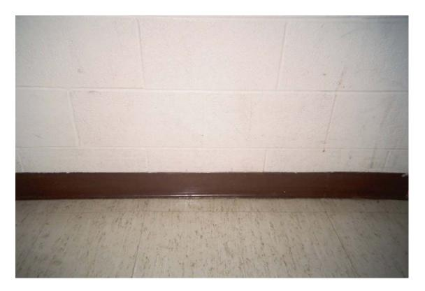
HA #7 – Non asbestos-containing 4" light brown cove molding and associated mastic
