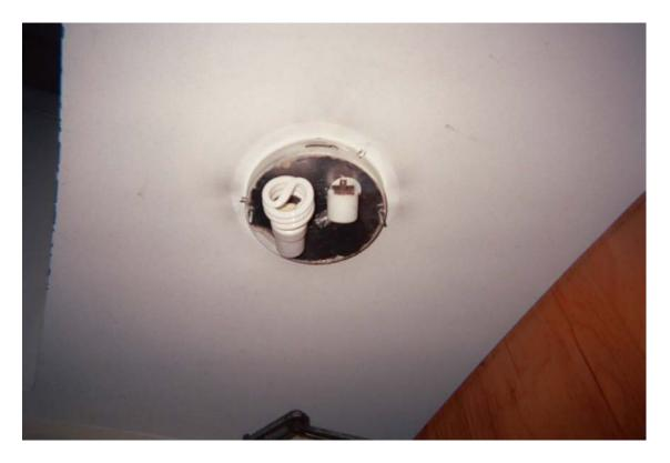
HA #40 – Asbestos-containing light heat shield insulation
