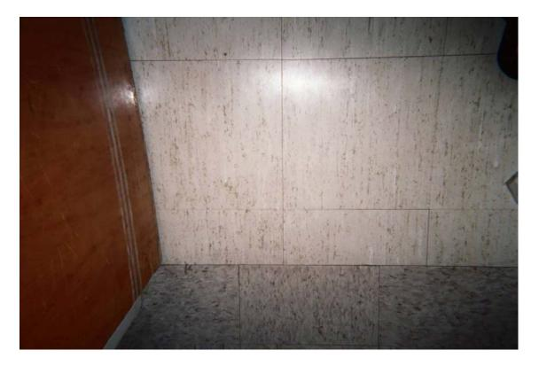
HA #11 – Non asbestos-containing 12" x 12" tan floor tile with marble pattern and associated asbestos-containing mastic
