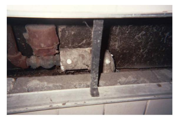
HA #19 – Asbestos-containing steam/condensate supply and return pipe straight insulation
