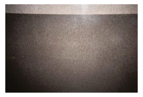
HA #37 – Non asbestos-containing 12" x 12" dark gray floor tile with marble pattern and associated asbestos-containing mastic
