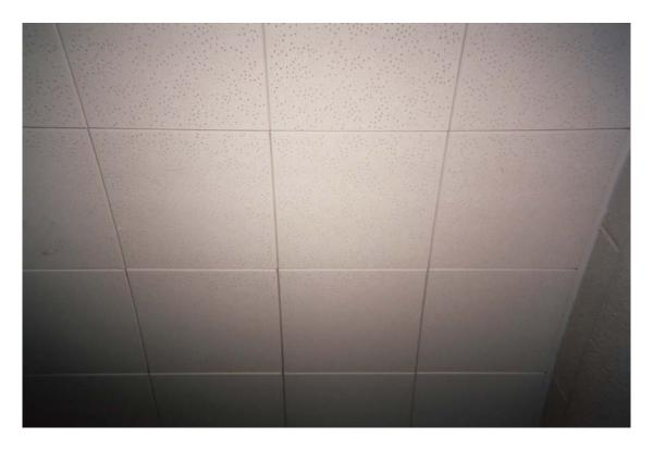
HA #6 – Non asbestos-containing 12" x 12" white ceiling tile with pin holes and associated glue pods
