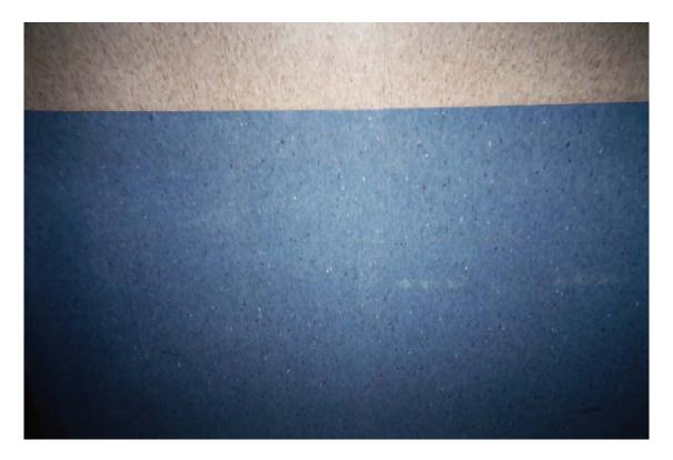
HA #36 – Non asbestos containing 12" x 12" blue floor tile with marble pattern and associated asbestos-containing mastic
