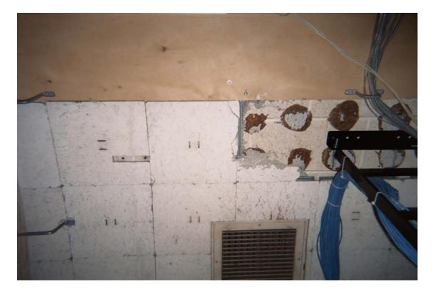
HA #32 – Non asbestos-containing 12" x 12" white spline ceiling tile with pin holes and fissures and associated glue pods
