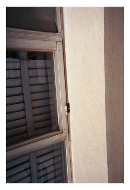
HA #26 – Assumed asbestos-containing window and door frame caulk compound
