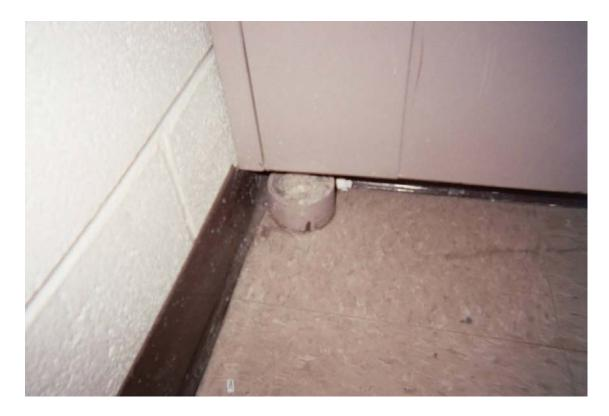
HA #33 – Non asbestos-containing gray pipe chase mud packing compound
