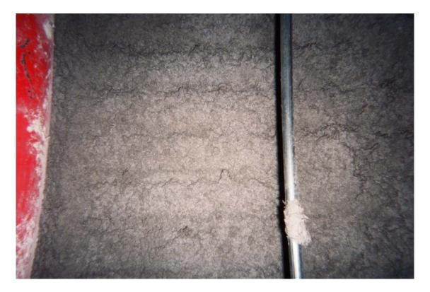
HA #1 – Non asbestos-containing spray-on fireproofing
