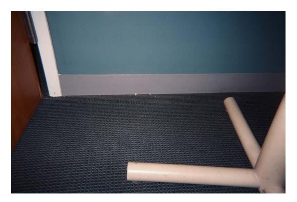
HA #41 – Non asbestos-containing 4" gray cove molding and associated mastic
