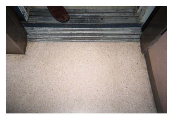
HA #10 – Non asbestos-containing tan vinyl flooring with blue specks and associated mastic
