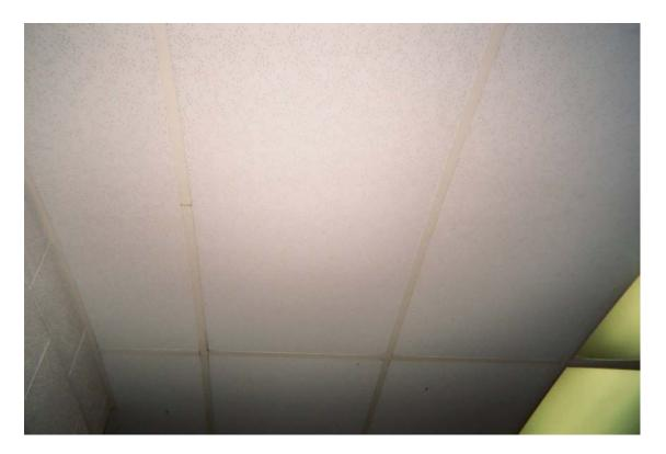
HA #30 – Non asbestos-containing 2' x 4' white lay-in ceiling tile with pin holes
