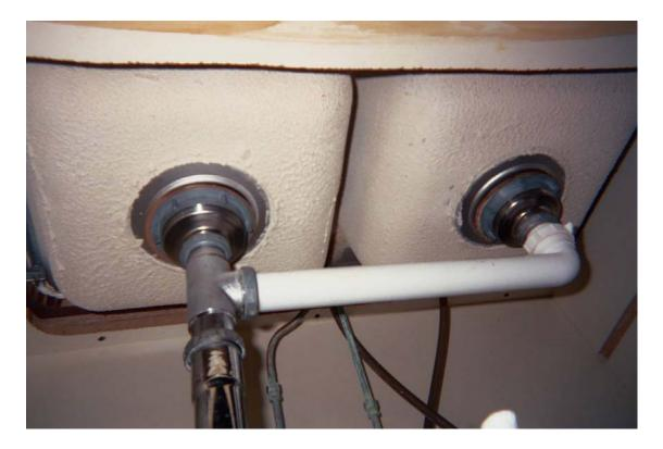
HA #38 – Non asbestos-containing white sink undercoating.
