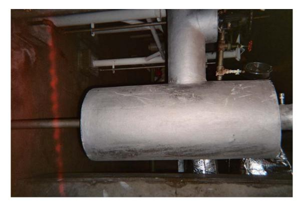
HA #22 - Asbestos-containing hot water heating expansion tank insulation
