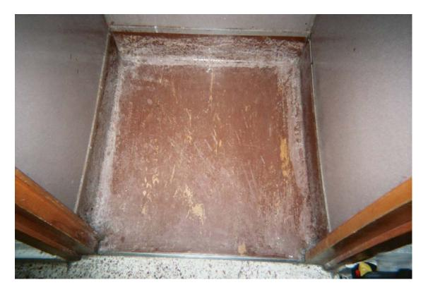
HA #13 – Non asbestos-containing brown linoleum flooring with rust streaks and associated mastic
