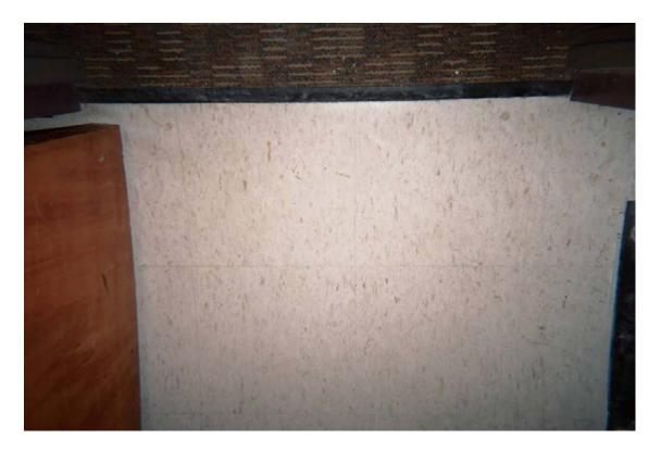
HA #12 – Non asbestos-containing 12" x 12" cream floor tile with white and green streaks and associated asbestos-containing mastic
