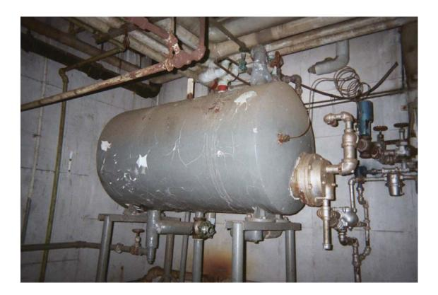
Asbestos-containing hot water holding tank insulation
