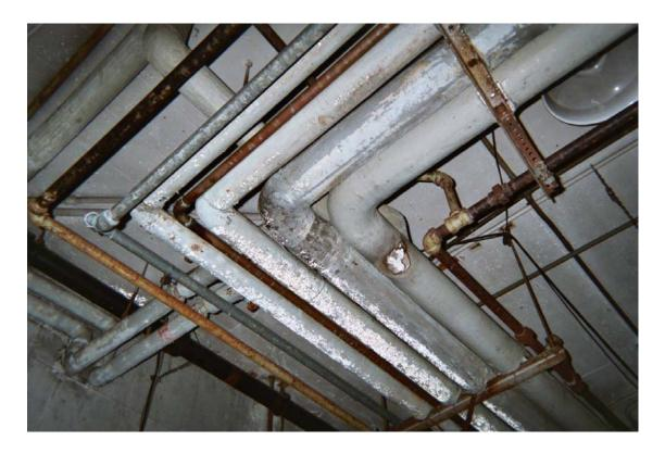
Asbestos-containing domestic water pipe joint and hanger insulation
