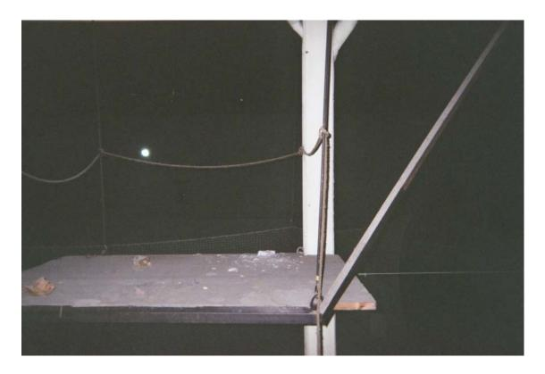
Asbestos-containing raised platform ACM debris
