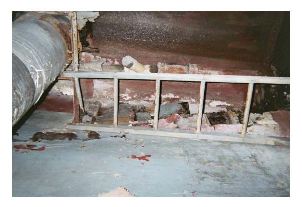
Asbestos-containing boiler thermal system insulation
