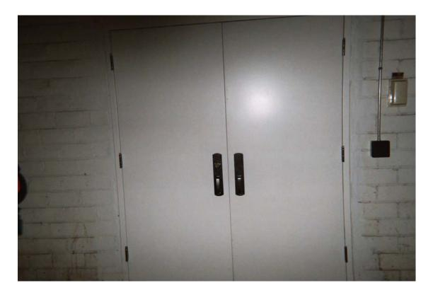
Assumed asbestos-containing fire door and frame
