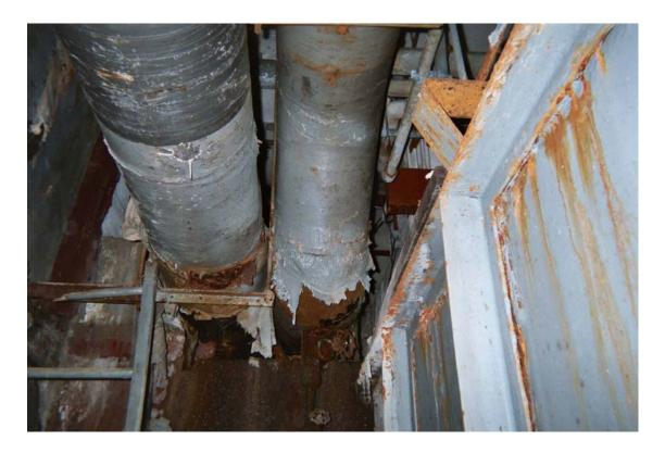
Asbestos-containing steam/condensate pipe straight insulation
