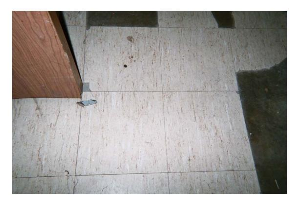
Asbestos-containing 9" x 9" wood grain pattern floor tile
