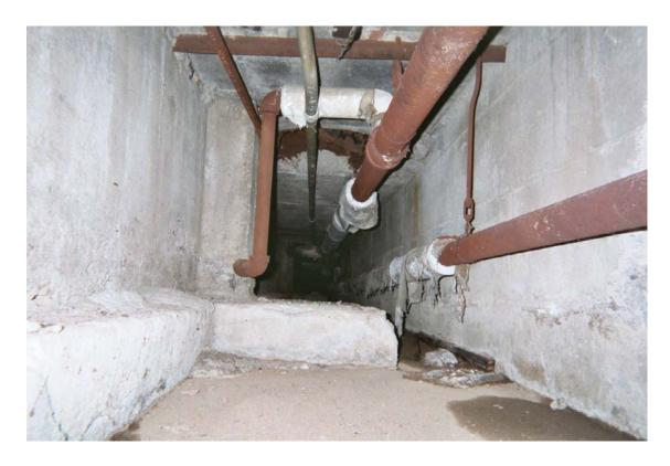
Asbestos-containing steam/condensate pipe straight insulation
