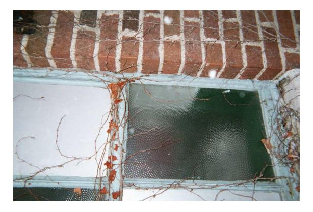
Assumed asbestos-containing window and door frame caulk compound
