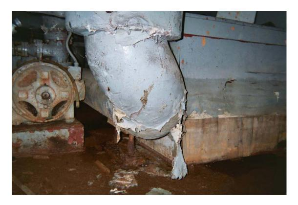
Asbestos-containing steam/condensate pipe joint and hanger insulation
