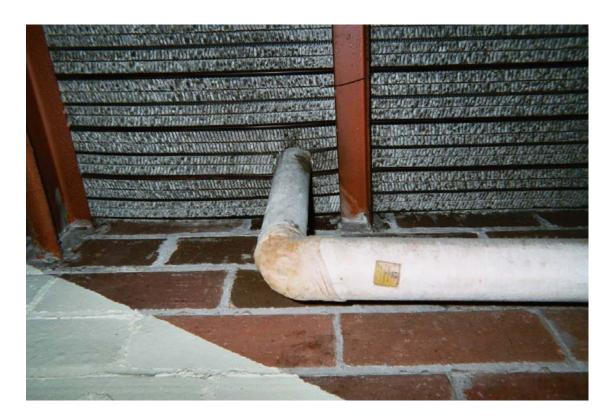
Asbestos-containing steam/condensate pipe straight insulation
