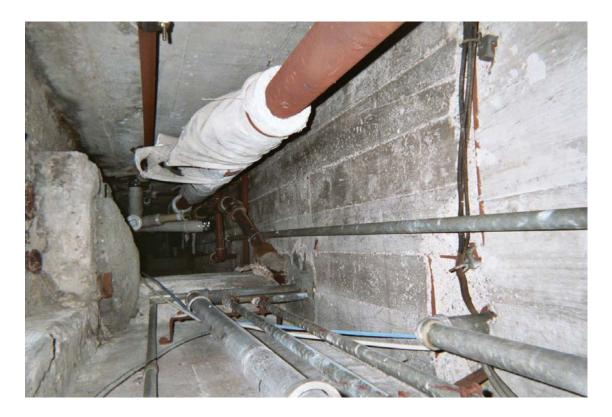
Asbestos-containing steam/condensate pipe straight insulation
