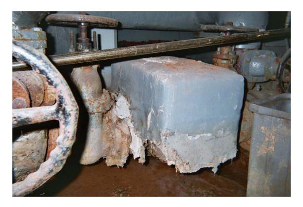
Damaged thermal system insulation, Boiler Room
