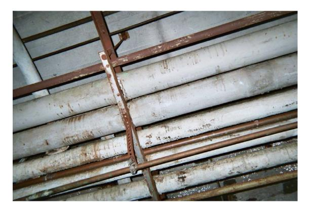
Asbestos-containing domestic water pipe straight insulation
