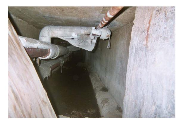
Asbestos-containing steam/condensate pipe joint and hanger insulation
