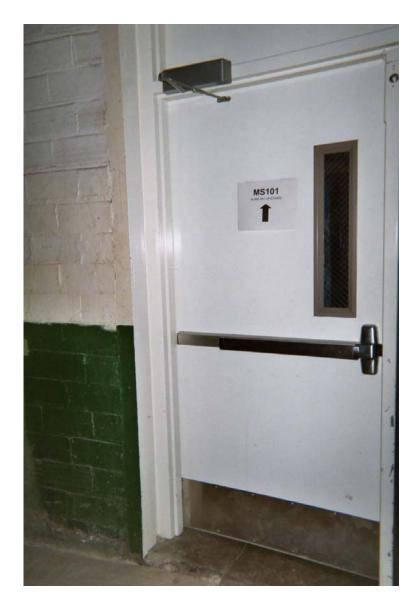
Assumed asbestos-containing fire door and frame
