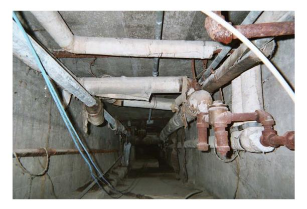
Asbestos-containing steam/condensate pipe straight insulation
