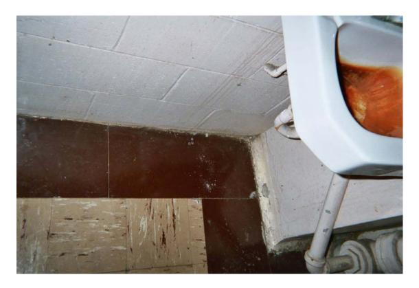
Asbestos-containing 1' x 2' brown floor tile
