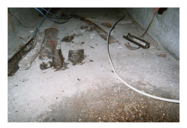
Asbestos-containing steam pipe straight insulation ACM debris on floor of tunnel area
