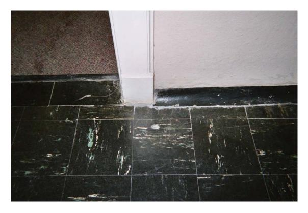
Asbestos-containing 9" x 9" black floor tile with cream and green streaks
