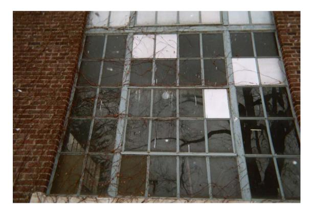
Assumed asbestos-containing window glazing compound
