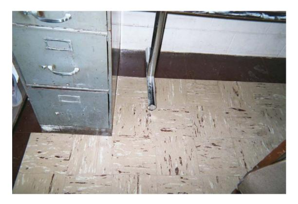
Asbestos-containing 9" x 9" tan floor tile with cream and rust streaks
