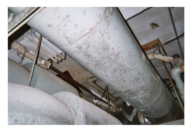
Asbestos-containing Steam/condensate pipe straight insulation
