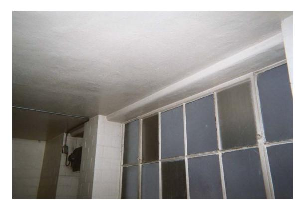
Assumed asbestos-containing window glazing compound
