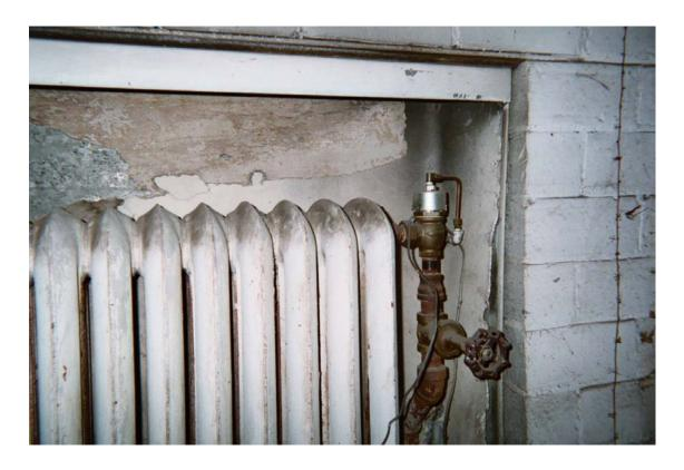
Asbestos-containing radiator backing paper
