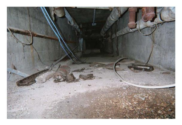
Asbestos-containing steam pipe straight insulation ACM debris on floor of tunnel area
