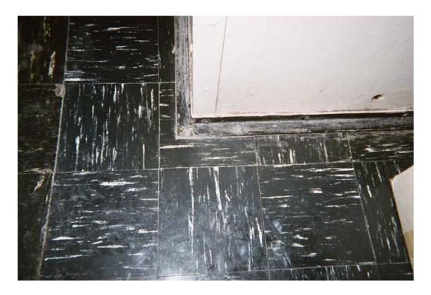
Asbestos-containing 9" x 9" black floor tile with cream streaks
