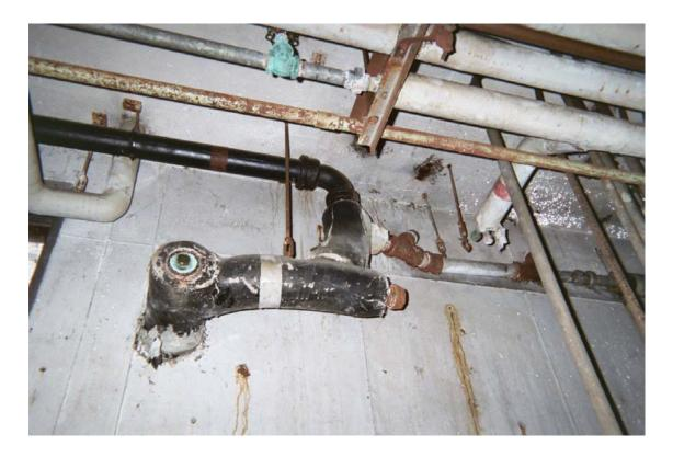
Asbestos-containing sewer drain pipe straight insulation and asbestos-containing sewer drain pipe joint and hanger insulation
