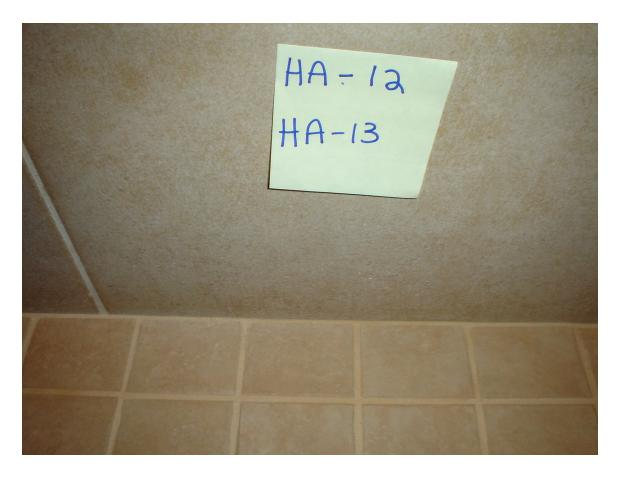
HA #12 – Non asbestos containing 2" x 2" light brown ceramic floor tile bedding compound
