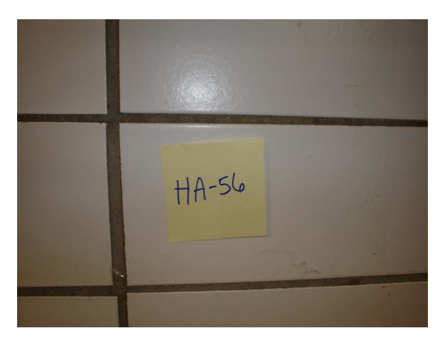
HA #56 – Non asbestos containing white ceramic wall tile bedding compound
