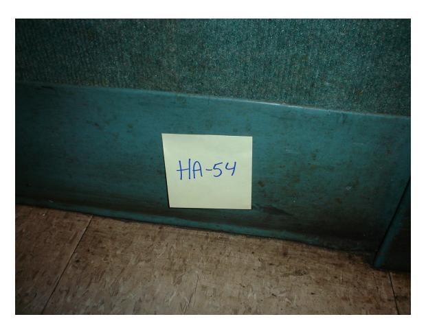
HA # 54 – Non asbestos containing 6" green cove molding and associated mastic
