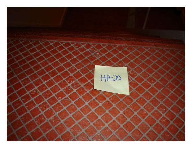
HA #20 – Asbestos containing red stair tread and associated non asbestos containing mastic
