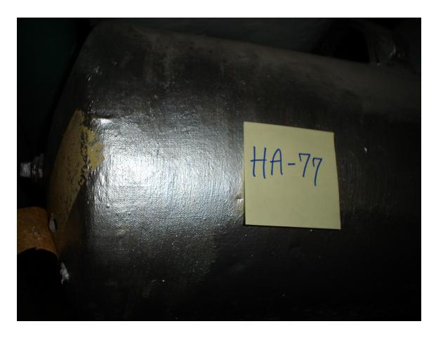
HA #77 – Asbestos containing tank insulation
