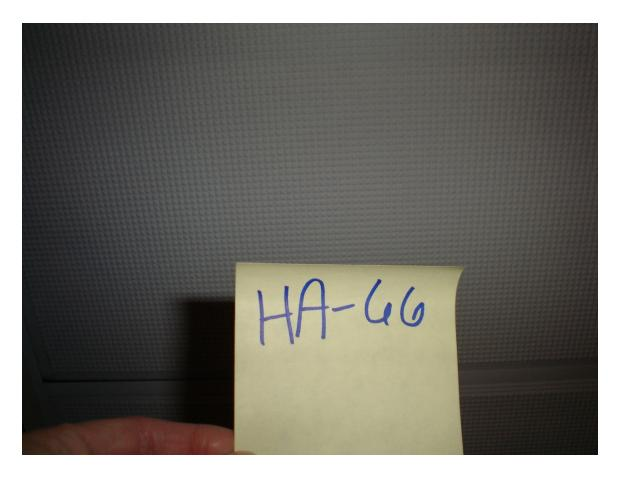
HA #66 – Non asbestos containing 2' x 2' white drop-in ceiling tile with tiny squares
