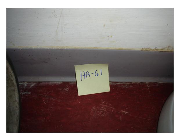
HA #61 – Non asbestos containing 4" gray cove molding and associated mastic
