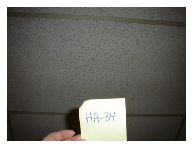
HA #34 – Non asbestos containing 2' x 4' white drop in ceiling tile with pin holes and fissures
