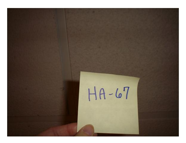
HA #67 – Non asbestos containing 2' x 2' white small textured drop ceiling tile
