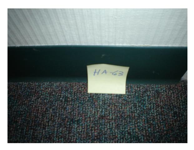
HA #63 – Non asbestos containing 4" green cove molding and associated mastic
