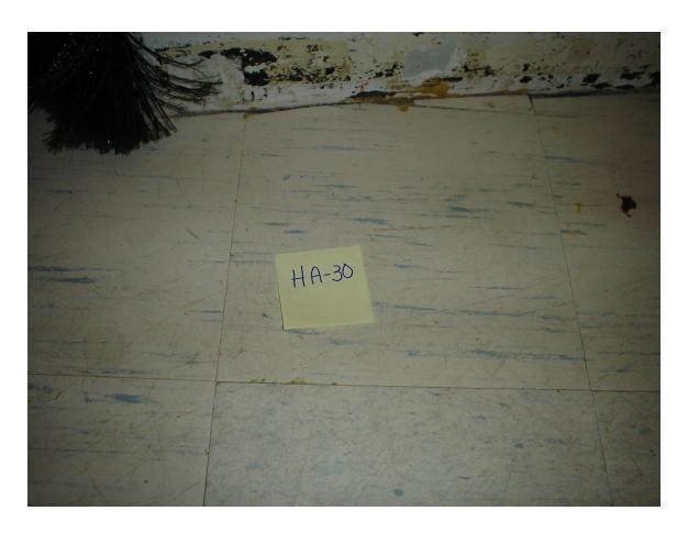
HA #30 – Non asbestos containing white floor tile with blue streaks and associated mastic
