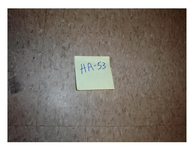
HA #53 – Non asbestos containing 12" x 12" beige floor tile with marble pattern and associated mastic
