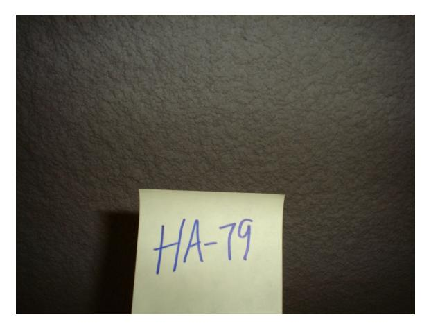
HA #79 – Non asbestos containing white acoustical ceiling
