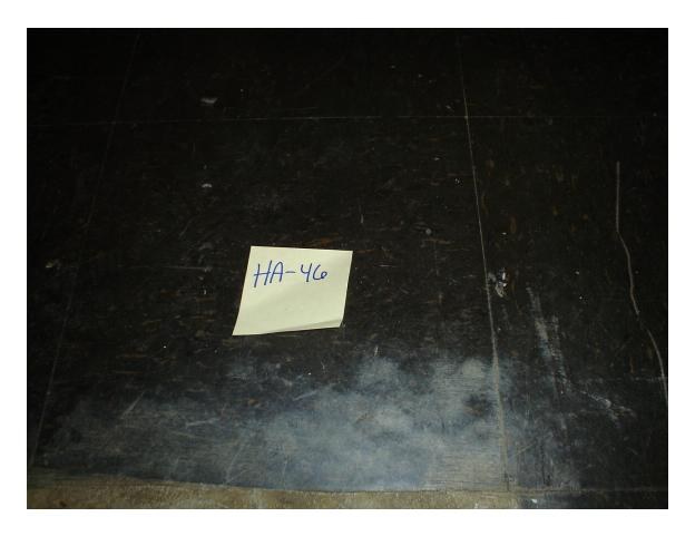
HA #46 – Asbestos containing 12" x 12" black floor tile with brown streaks and associated mastic
