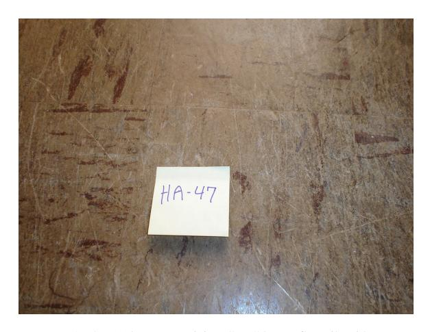
HA #47 – Asbestos containing 9" x 9" brown floor tile with brown and white streaks and associated non asbestos containing mastic
