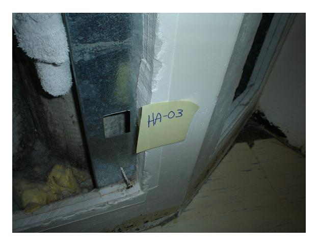
HA #3 – Non asbestos containing drywall with plaster skim coat
