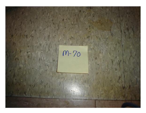
HA #70 – Non asbestos containing 12" x 12" gray floor tile with marble pattern and associated mastic
