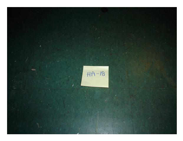
HA #18 – Non asbestos containing 12" x 12" green floor tile with white and black streaks and associated mastic
