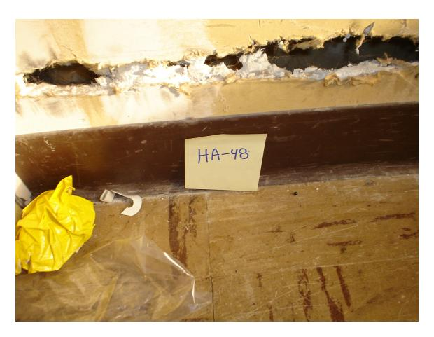
HA #48 – Non asbestos containing 4" dark brown cove molding and associated mastic
