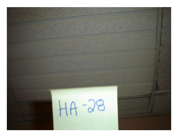
HA # 28 - Non asbestos containing 2' x 2' white lined drop ceiling tile
