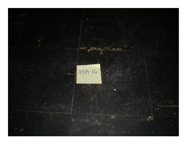
HA #16 – Asbestos containing 9" x 9" black floor tile with white streaks and associated non asbestos containing mastic
