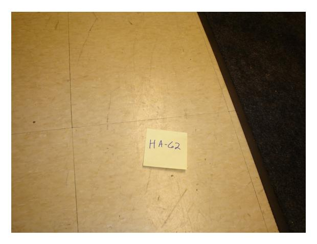
HA #62 – Non asbestos containing 12" x 12" white floor tile with brown and white streaks and associated asbestos containing mastic
