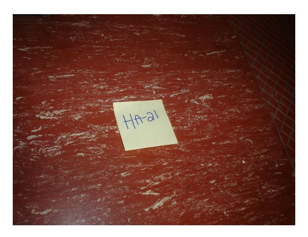
HA #21 – Non asbestos containing red linoleum with white streaks
