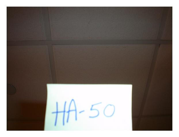
HA #50 – Non asbestos containing 2' x 2' white drop in ceiling tile with pin holes
