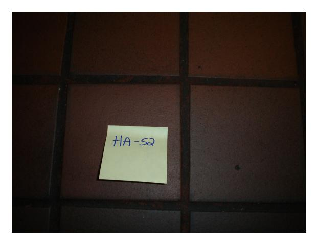
HA #52 – Non asbestos containing red ceramic floor tile with squares bedding compound
