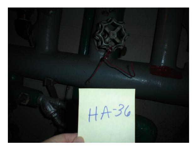
HA #36 – Asbestos containing steam pipe joint insulation
