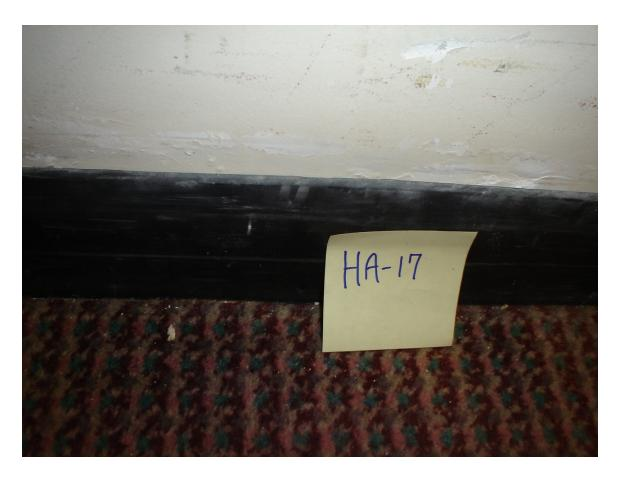
HA #17 – Non asbestos containing black cove molding and associated mastic
