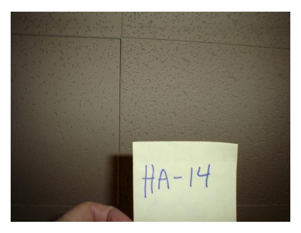
HA #14 – Non asbestos containing 12" x 12" light brown textured glued-on ceiling tile and associated glue pods
