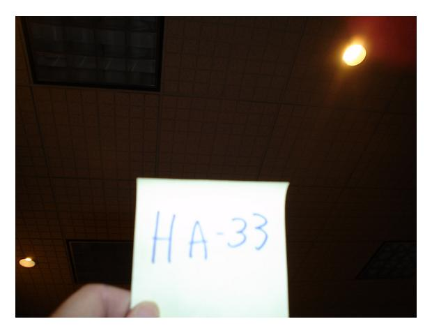
HA #33 – Non asbestos containing 2' x 2' white lay-in ceiling tile with raised 2" x 2" squares
