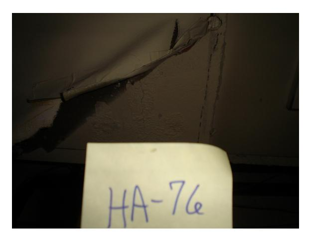
HA #76 – Non asbestos containing duct insulation
