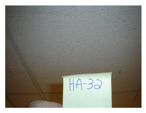
HA #32 – Non asbestos containing 2' x 2' white lay-in ceiling tile with pin holes and fissures
