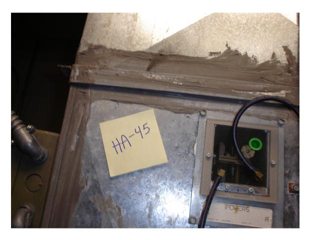
HA #45 – Non asbestos containing gray duct caulk
