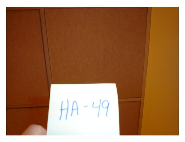
HA #49 – Non asbestos containing 2' x 2' off-white fuzzy drop-in ceiling tile
