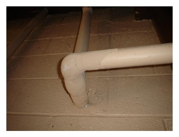
HA #2 – Non asbestos-containing domestic water supply pipe joint insulation (on fiberglass pipe straight insulation)
