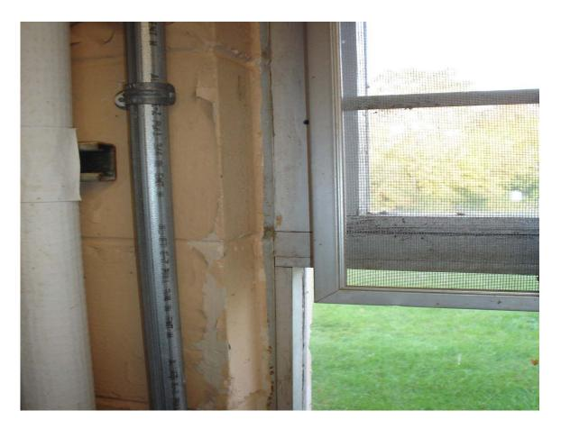
HA #1 – Asbestos-containing window and door frame caulk compound (interior)
