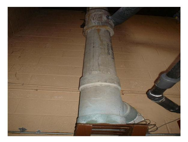
HA #5 – Asbestos-containing transite heat vent pipe
