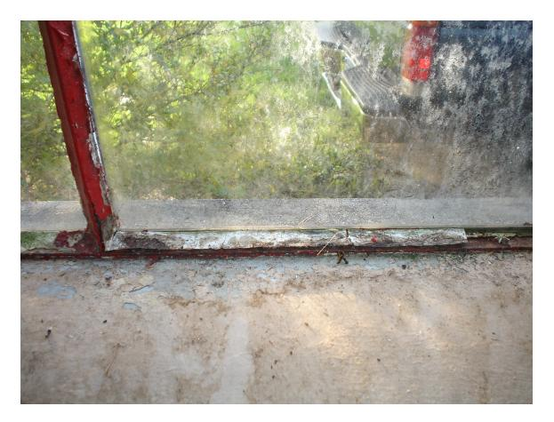
HA #3 – Asbestos-containing window glazing compound
