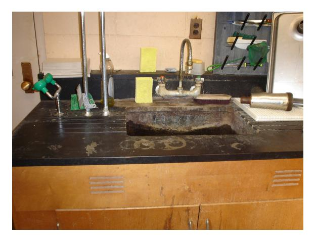
HA #4 – Assumed asbestos-containing laboratory sinks and table tops
