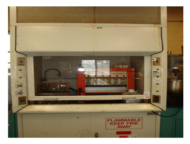
HA #6 - Assumed asbestos-containing laboratory fume hood
