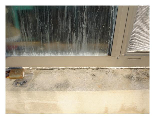
HA #8 – Asbestos-containing window and door frame caulk compound (exterior)
