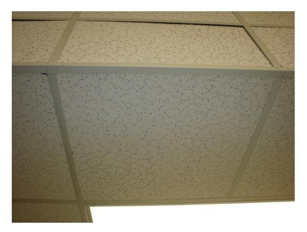
HA #3 – Non asbestos-containing 2' x 2' white lay-in ceiling tile with pin holes and fissures
