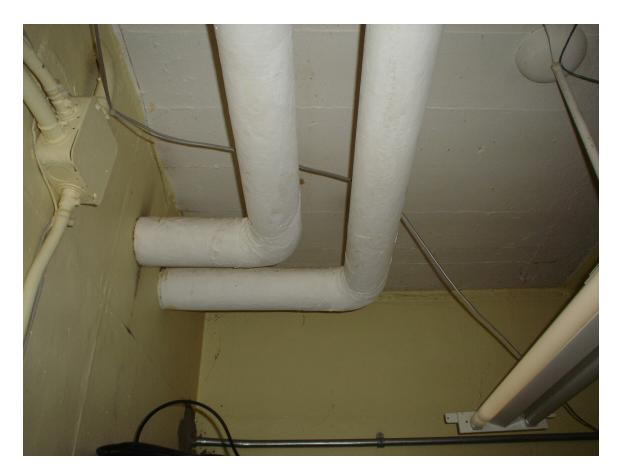
HA #8 – Asbestos-containing steam/condensate supply and return pipe joint insulation (on fiberglass line)
