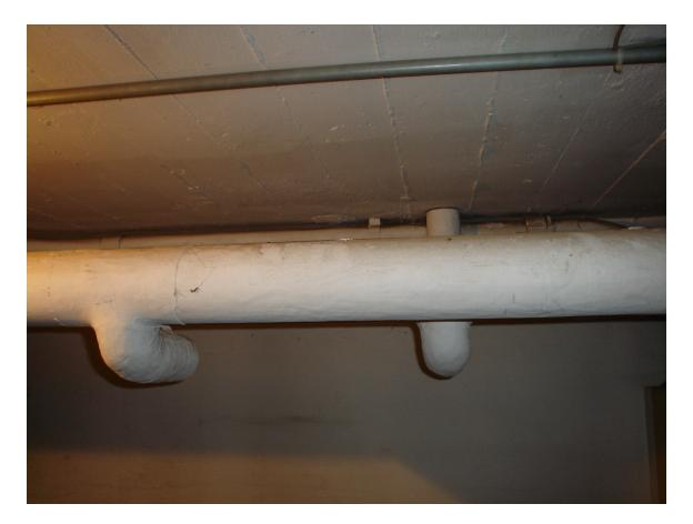
HA #7 – Non asbestos-containing steam/condensate supply and return pipe straight insulation (fiberglass line/canvas cover)
