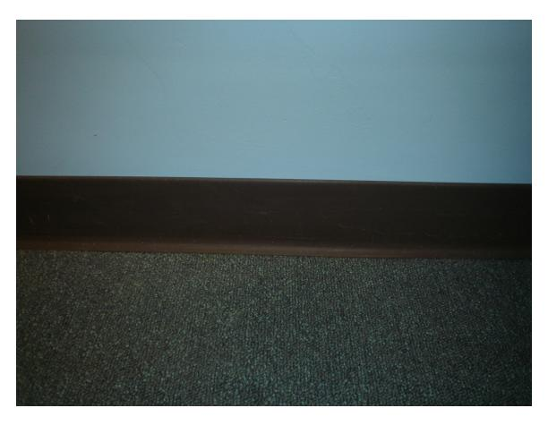
HA #4 – Non asbestos-containing 4" brown cove molding and associated mastic
