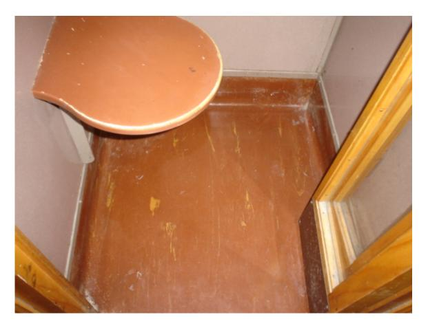
HA #46 – Non asbestos-containing red linoleum with rust streaks and associated backing
