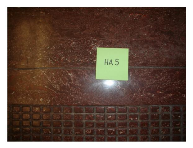
HA #5 – Asbestos-containing reddish linoleum flooring and stair tread with cream streaks and associated non asbestos-containing mastic
