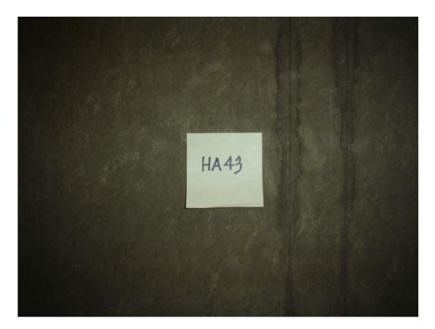
HA #43 – Assumed asbestos-containing transite wall panels
