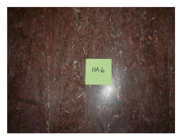
HA #6 – Asbestos-containing brown linoleum flooring and stair tread with cream and rust streaks and associated non asbestos-containing mastic
