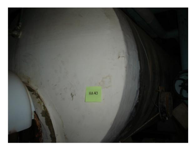
HA #40 – Asbestos-containing expansion tank insulation
