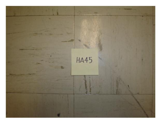
HA #45 – Asbestos-containing 9" x 9" white floor tile with green streaks and associated non asbestos-containing mastic
