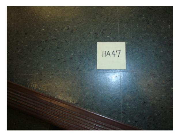
HA #47 – Non asbestos-containing 12" x 12" green floor tile with dark green and tan specks and associated mastic
