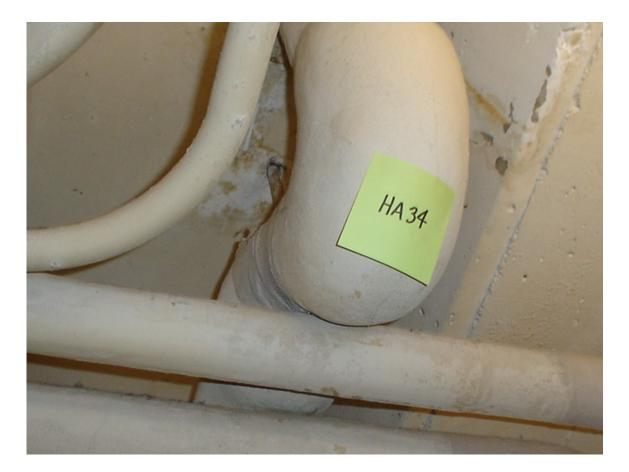
HA #34 – Asbestos-containing drain pipe joint and hanger insulation
