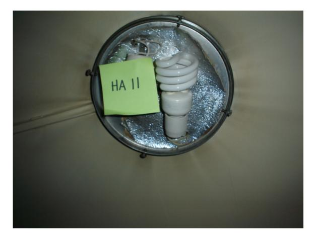
HA #11 – Asbestos-containing light heat shield
