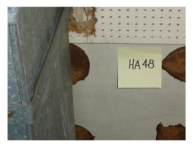
HA #48 – Non asbestos-containing 12" x 12" white ceiling tile with uniform holes and associated glue pods
