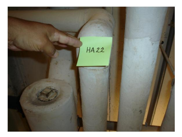
HA #22 – Asbestos-containing domestic water supply pipe joint and hanger insulation
