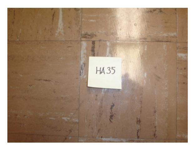
HA #35 – Asbestos-containing 9" x 9" light brown floor tile with cream and rust streaks and associated non asbestos-containing mastic
