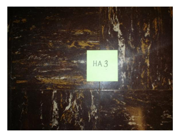
HA #3 – Asbestos-containing 9" x 9" brown floor tile with cream and rust streaks and associated mastic
