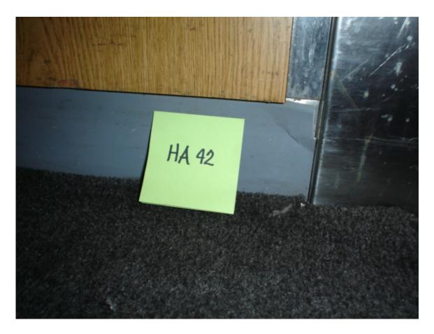
HA #42 – Non asbestos-containing 4" gray cove molding and associated mastic
