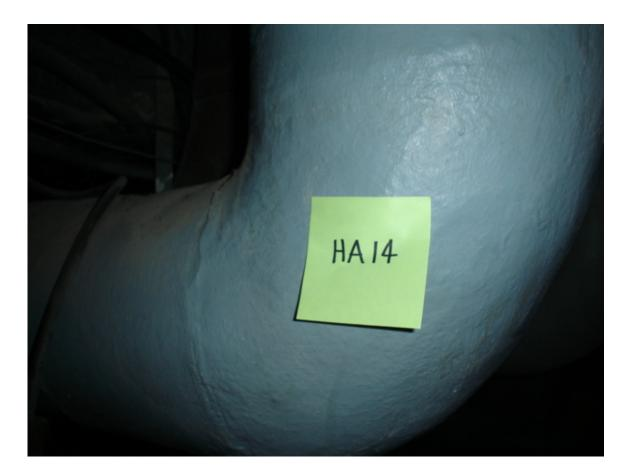
HA #14 – Asbestos-containing steam/condensate supply and return pipe joint and hanger insulation
