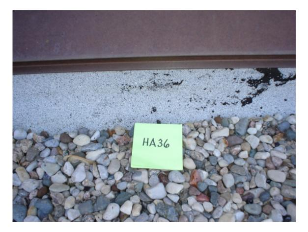
HA #36 - Assumed asbestos-containing roofing materials and products
