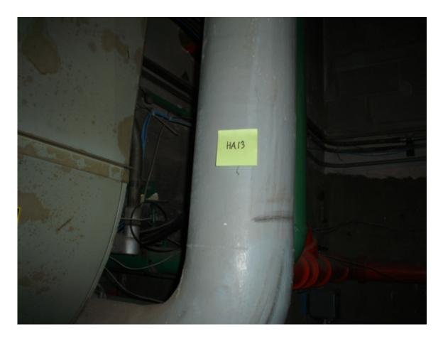
HA #13 – Asbestos-containing steam/condensate supply and return pipe straight insulation
