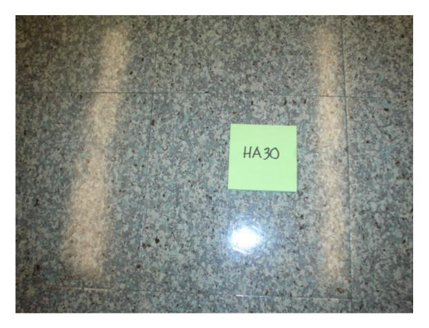
HA #30 – Asbestos-containing 9" x 9" gray floor tile with cream specks and associated mastic
