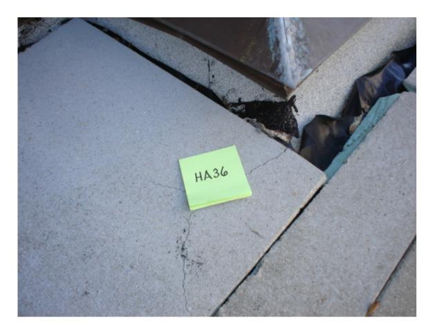
HA #36 - Assumed asbestos-containing roofing materials and products
