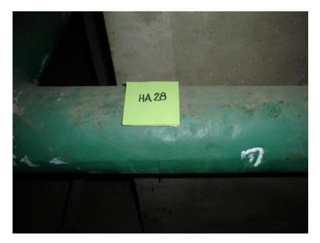
HA #28 – Asbestos-containing domestic water supply pipe straight insulation
