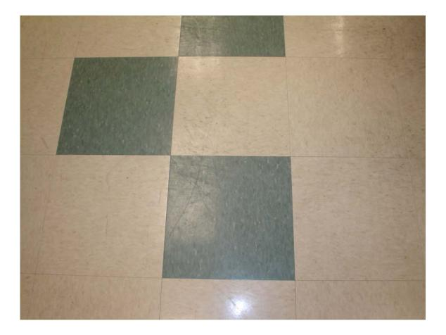
HA #22 – Non asbestos containing 12" x 12" blue marble pattern floor tile and associated mastic
