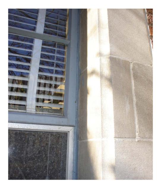
HA #46 – Assumed asbestos containing window and door frame caulk compound
