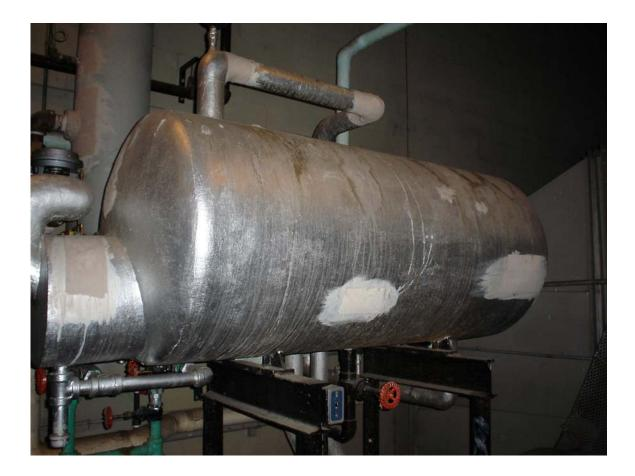
HA #7 – Asbestos containing hot water holding tank insulation
