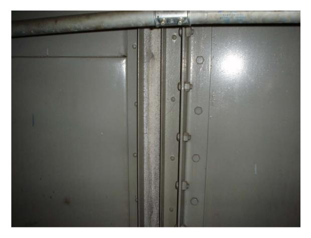
HA #8 – Asbestos containing ventilation duct expansion cloth
