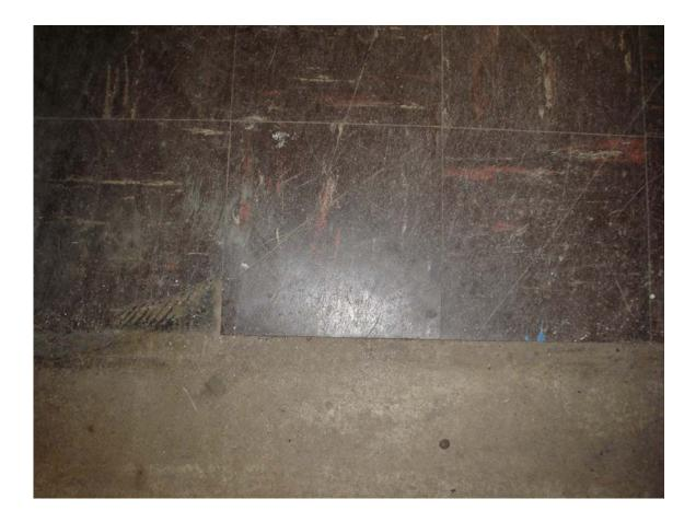
HA #10 – Asbestos containing 9" x 9" brown floor tile with cream and red streaks and associated non asbestos containing mastic
