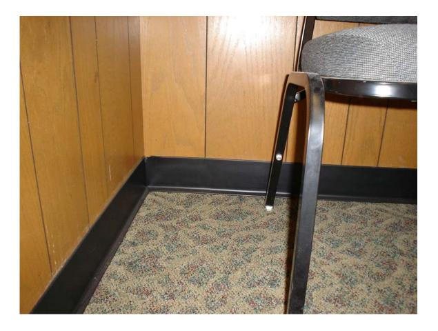
HA #13 – Non asbestos containing 4" black cove molding and associated mastic
