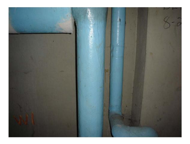
HA #3 – Non asbestos containing domestic water supply pipe straight insulation
