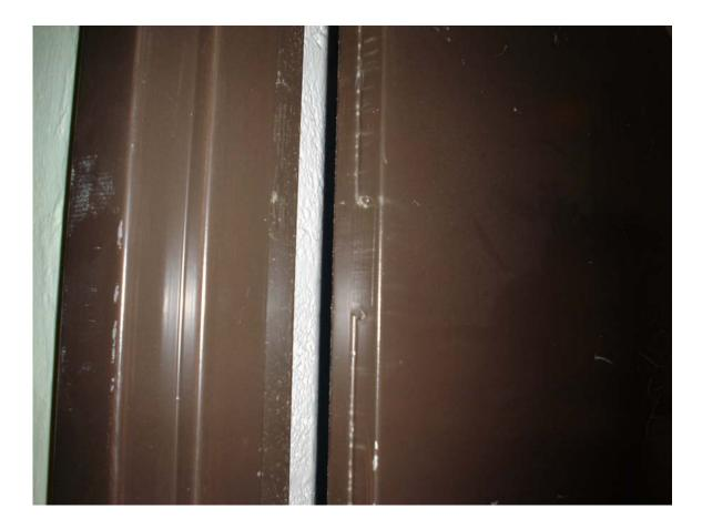
HA #20 – Assumed asbestos containing fire door and frame
