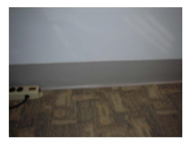
HA #23 – Non asbestos containing 6" gray cove molding and associated mastic
