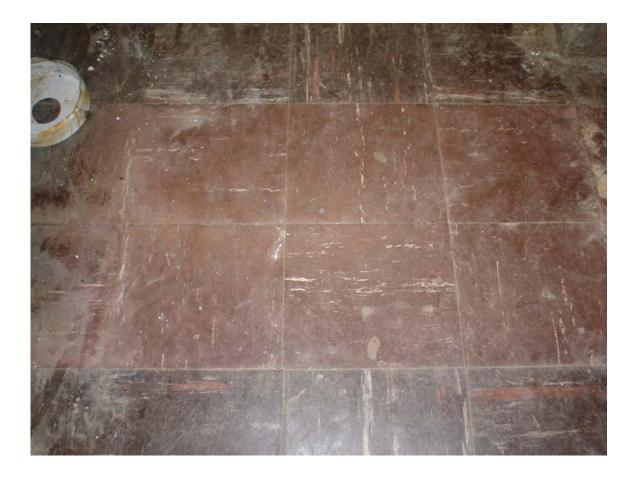
HA #11 – Asbestos containing 9" x 9" rust floor tile with cream and red streaks and associated non asbestos containing mastic
