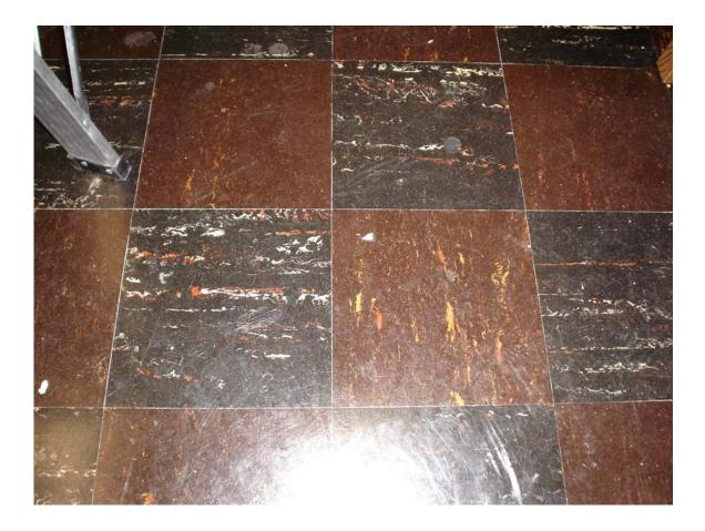
HA #31 – Asbestos containing 12" x 12" black floor tile with cream and red streaks and associated non asbestos-containing mastic
