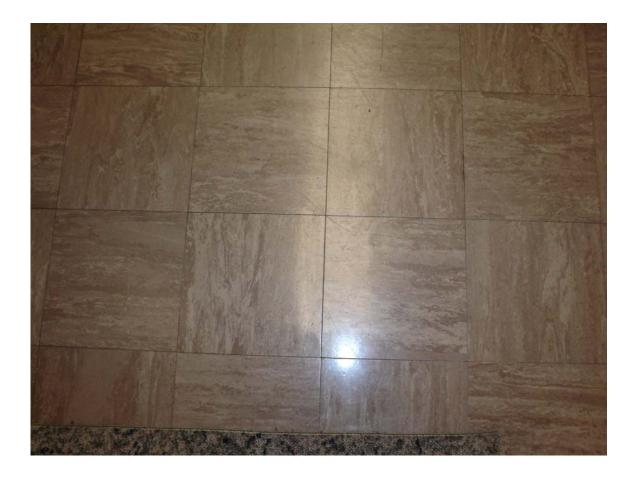
HA #29 – Asbestos containing 9" x 9" tan floor tile with swirl pattern and associated non asbestos containing mastic
