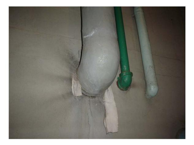
HA #6 – Asbestos containing steam/condensate supply and return pipe joint and hanger insulation
