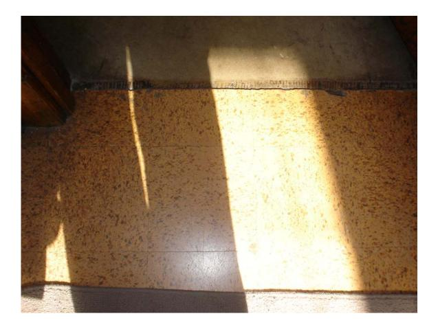
HA #44 – Asbestos containing 9" x 9" brown floor tile with multi-colored brown speckles and non asbestos containing associated mastic
