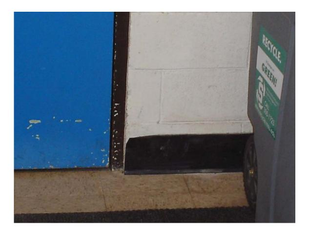
HA #9 – Asbestos containing 6" black cove molding and associated non asbestos containing mastic
