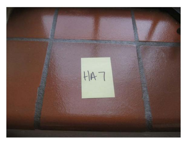
HA #7 – Assumed asbestos containing Orange ceramic tile and associated bedding compound
