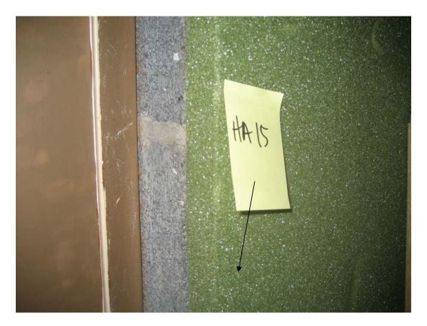
HA #15 –asbestos containing black gluepods on Green soundproofing (Green soundproofing NON-ACM)
