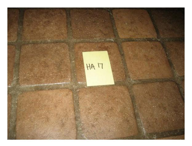
HA #17 – Assumed asbestos containing 2"x 2" Brown ceramic tile and bedding compound
