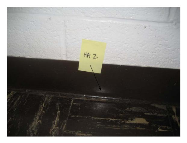
HA #2 – Non asbestos containing 4" Brown cove molding and associated mastic
