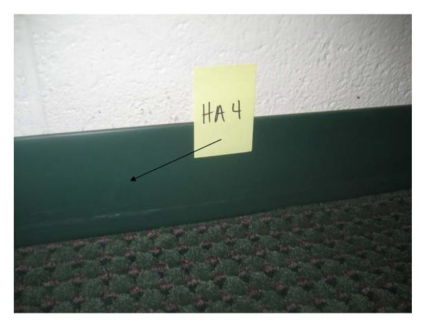
HA #4 – Non asbestos containing 4" Green cove molding and associated mastic
