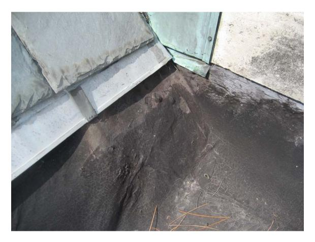
HA #21 – Assumed asbestos containing Roofing materials and products
