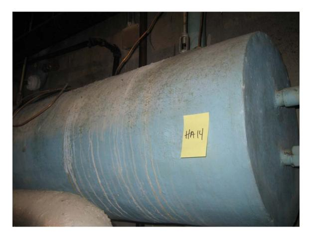
HA #14 – Asbestos containing Mag tank insulation
