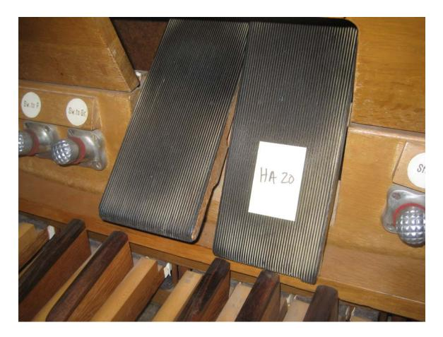
HA #20 – Assumed asbestos containing Black vinyl pedal tread and associated mastic
