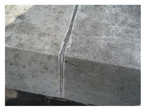
HA #22 – Assumed asbestos containing Light gray masonry caulk
