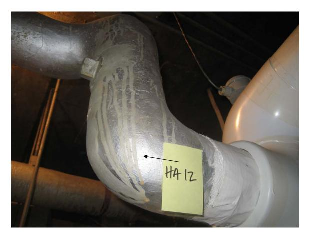
HA #12 – Asbestos containing pipe joint and hanger insulation
