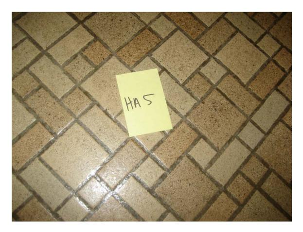
HA #5 – Assumed asbestos containing Multi shade and size brown ceramic tile and bedding compound
