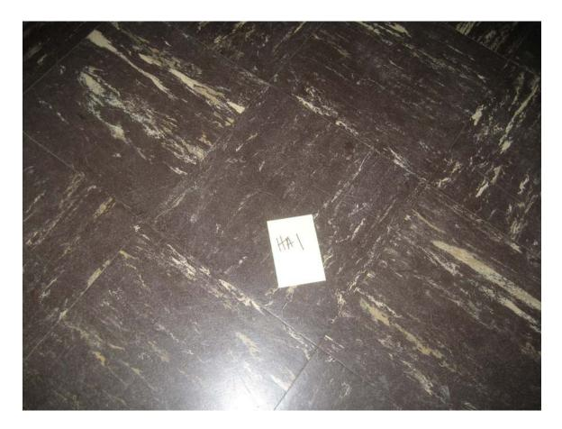
HA #1 –Asbestos containing 9"x 9" Dark brown floor tile with white and cream streaks (mastic negative)
