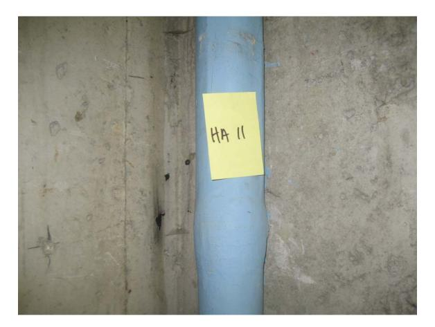
HA #11 – Asbestos containing Straight pipe insulation
