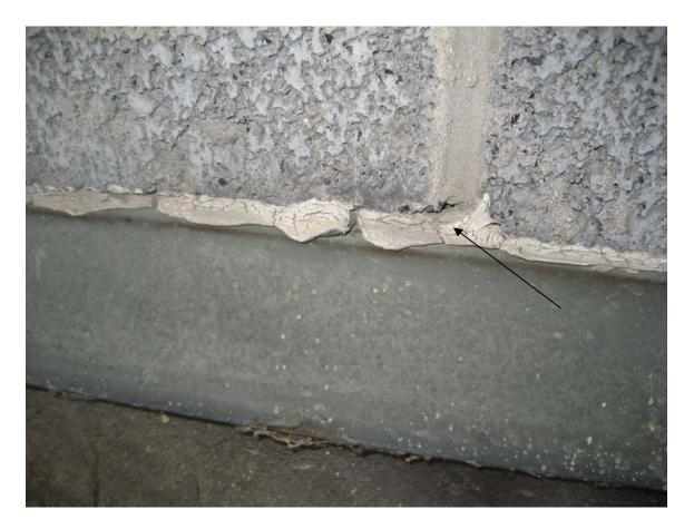
HA #23 – Asbestos containing White bell tower building caulk
