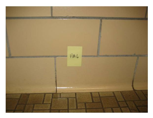
HA #6 – Assumed asbestos containing Tan ceramic wall tile and associated bedding compound
