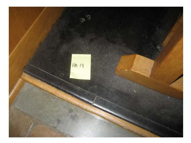
HA #19 – Assumed asbestos containing black vinyl sheet flooring and associated mastic
