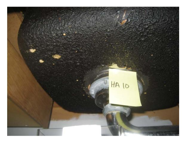
HA #10 –Asbestos containing Black sink undercoating
