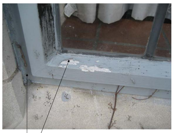
HA #24 – Assumed asbestos containing White window glazing HA #25 – Assume asbestos containing White window caulk
