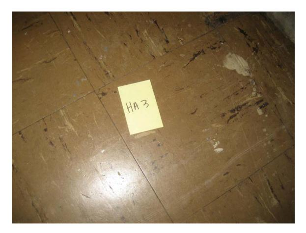
HA #3 – Asbestos containing 9"x 9" Light brown floor tile with white and black streaks (mastic negative)
