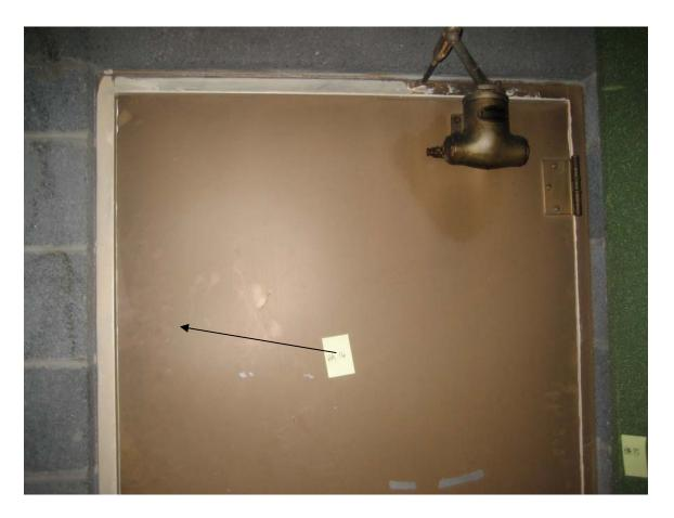
HA #16 – Assumed asbestos containing Fire door and frames
