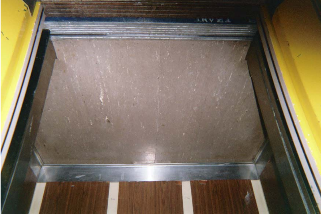
Photo 10 – Non asbestos-containing tan linoleum with cream and black streaks
