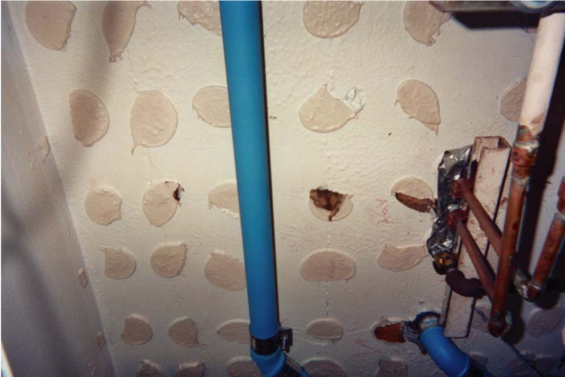
Photo 2 – Non asbestos-containing ceiling glue pods
