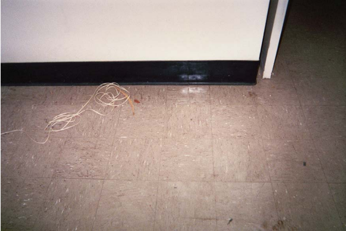
Photo 3 – Asbestos-containing 9” x 9” gray floor tile with white and rust streaks
