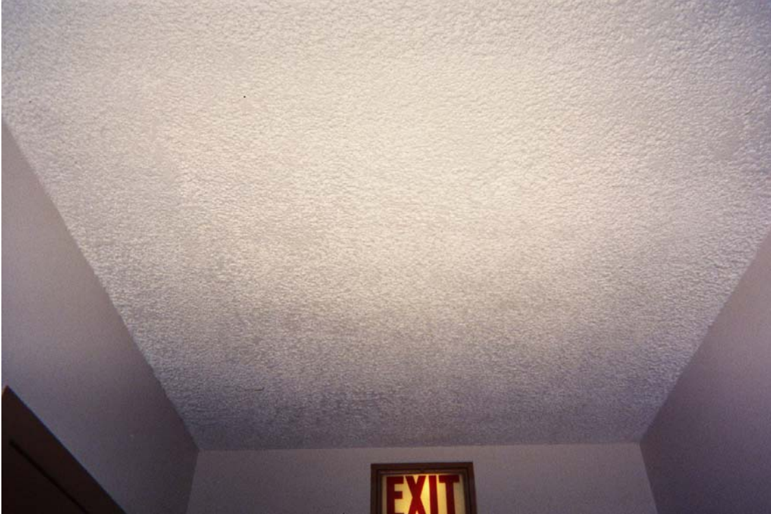
Photo 1 – Non asbestos-containing spray-on acoustical ceiling plaster
