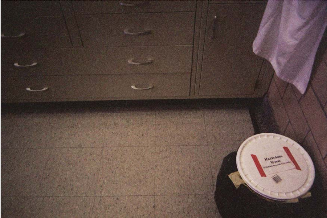
Photo 6 – Asbestos-containing 9” x 9” tan floor tile with cream, pink and brown streaks
