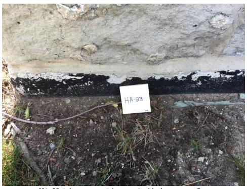
HA-23 Asbestos containing exterior black waterproofing
