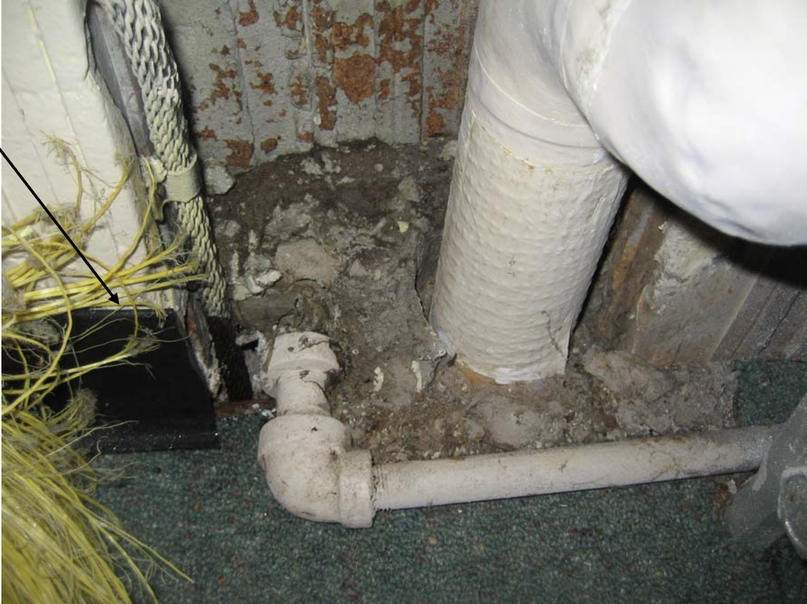
HA #2 – Non asbestos containing 4” black cove molding and associated mastic
