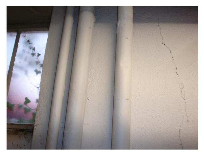
HA #9 – Asbestos-containing domestic water supply pipe straight insulation
