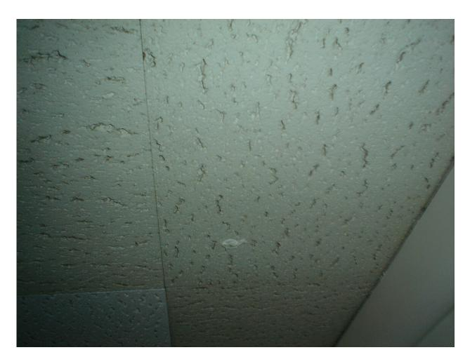
HA #16 – Non asbestos-containing 12" x 12" white ceiling tile with fissures and associated glue pods
