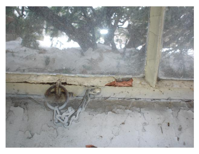
HA #5 – Non asbestos-containing window glazing caulk compound
