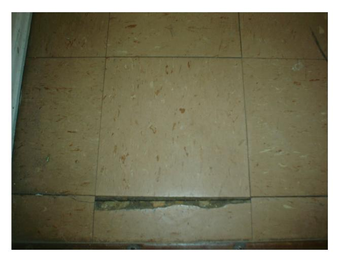
HA #6 – Asbestos-containing 9" x 9" tan floor tile with cream and tan streaks and associated non asbestos-containing mastic
