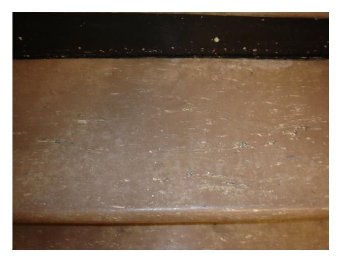
HA #7 – Asbestos-containing brown linoleum with cream and black streaks and associated non asbestos containing mastic
