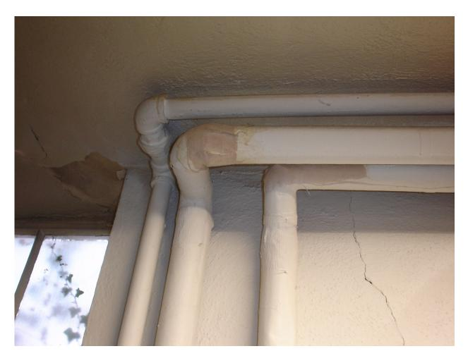
HA #10 – Asbestos-containing domestic water supply pipe joint and hanger insulation
