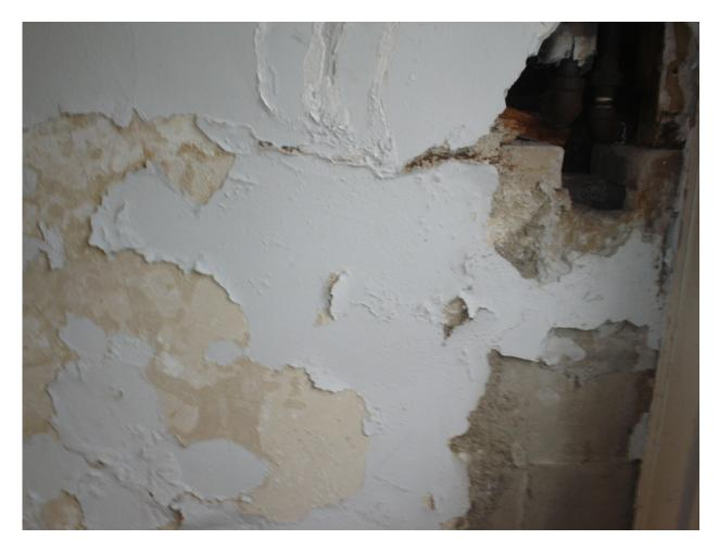
HA #3 – Asbestos-containing smooth wall and ceiling plaster
