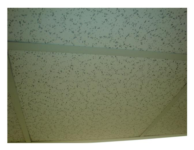
HA #12 – Non asbestos-containing 2' x 2' white lay-in ceiling tile with pin holes and fissures
