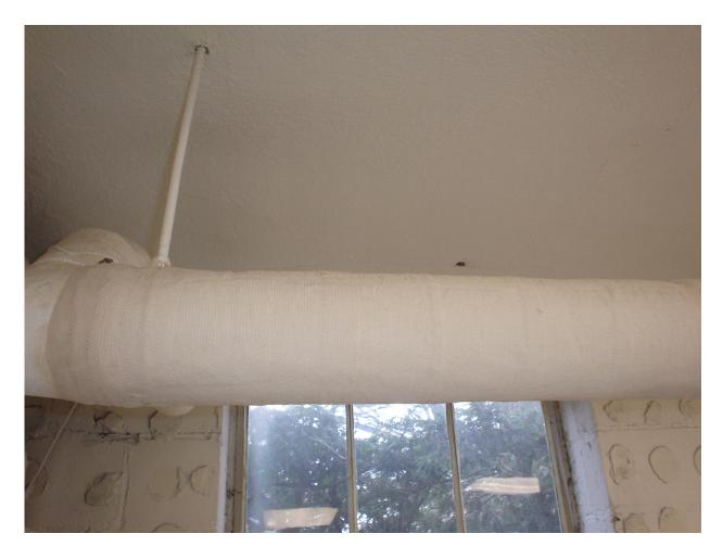
HA #1 – Asbestos-containing steam and condensate supply and return pipe straight insulation
