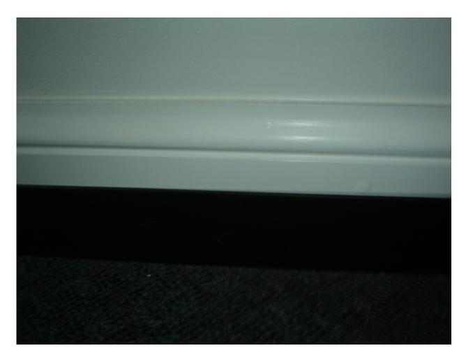
HA #14 – Non asbestos-containing 4" black cove molding and associated mastic
