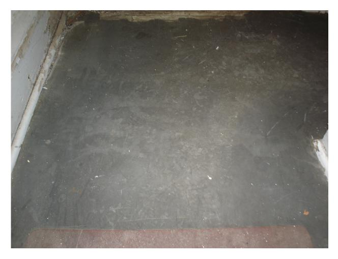
HA #8 - Non asbestos-containing dark green linoleum and associated mastic
