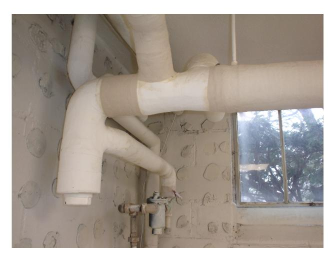
HA #2 – Asbestos-containing steam and condensate supply and return pipe joint and hanger insulation
